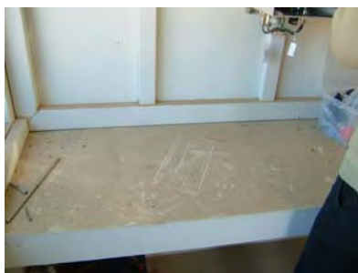
Rainfall Gauging Station (before)
