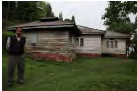
Dilapidated office of Territorial Circle
