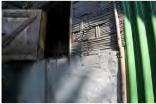
Forest guard's residence with traditional structure reinforced by bamboo
