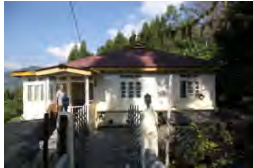
Old building of Forest Guard's residence
