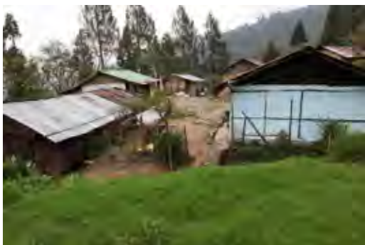
Old and dilapidated staff quarters
