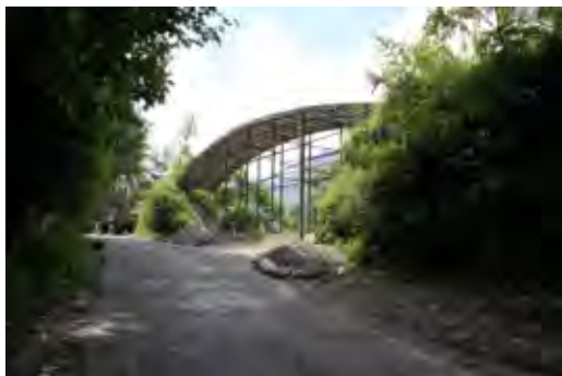
Butterfly park under construction (near Mangan)
