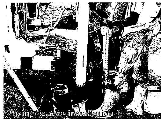
Inspection of casing screen
