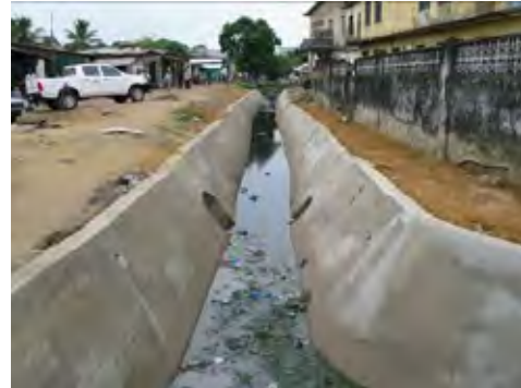
Upgraded in February 2008
