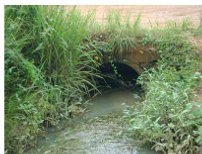
BS-06 -Island Clinic Road Culvert Island Clinic Community
