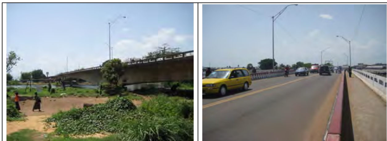
Figure 4.3-5 Present Situation of Johnson Street Bridge
