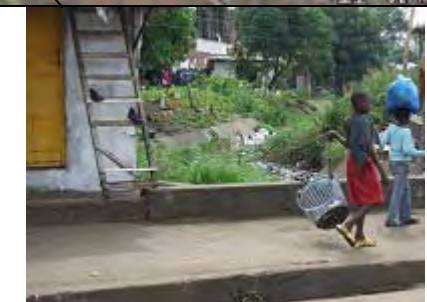
Drainage in Soniwein community crosses Lynch Street
