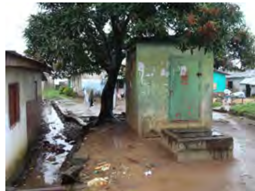
Figure 2.6-8 Slipway P.S to Lift Up Sewage to the Manhole
