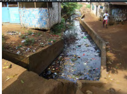
Open channel of concrete lining crosses Russell Avenue in Jallah Community
