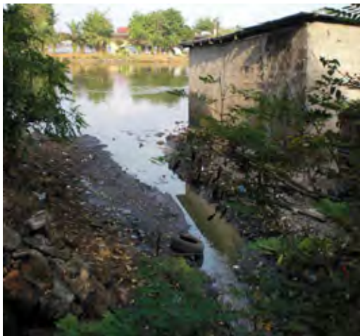
Figure 2.6-5 Sewage is Discharged into Mesurado River from Pump Station
