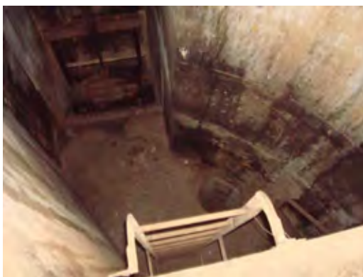
Figure 2.6-7 Underground Pit in BTC P.S
