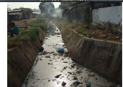
Soniwein drainage crosses Randell Street
