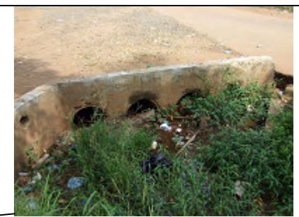
4 set pipe culverts of Coleman Avenue at 18th Street. Flow capacity is less by siltation.
