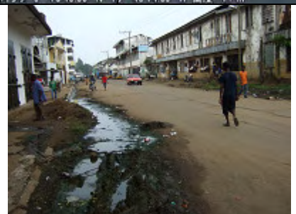
Road side gutter in West Point Road. It is covered by mud and garbage.
