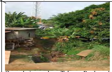
Cross drainage along Tubman Boulevard near Hospital
