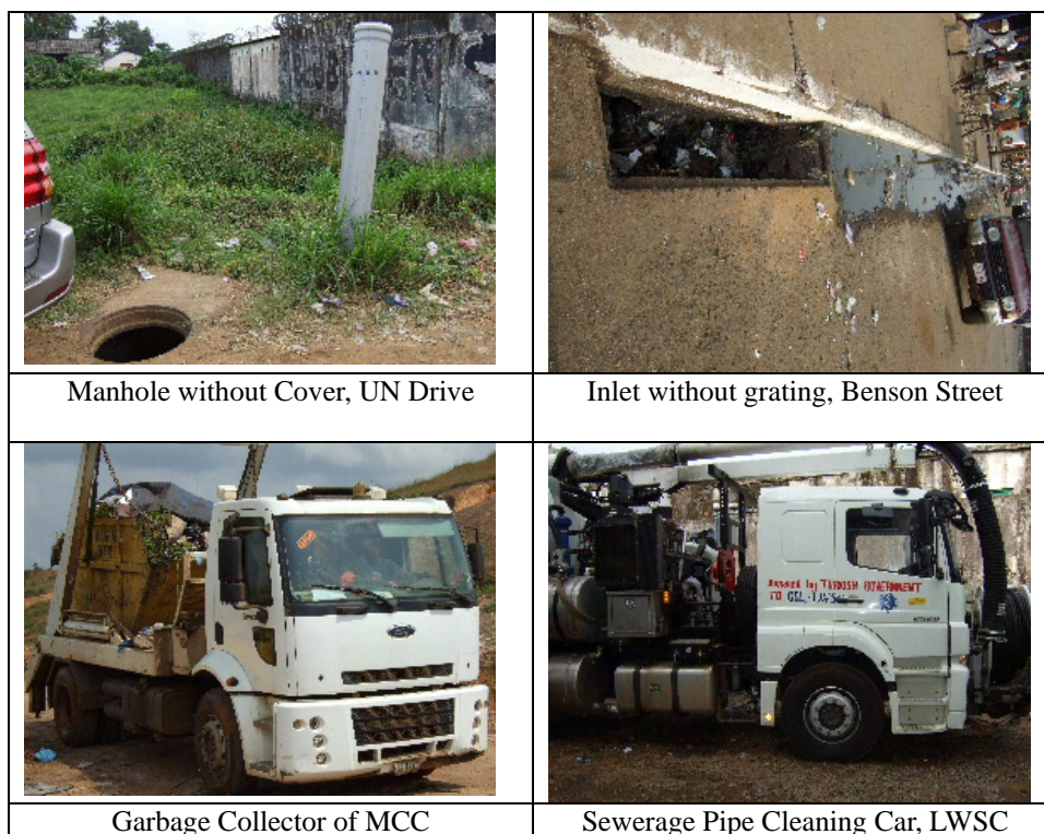
Figure 2.7-4 Present Condition of Drainage Structure and Equipment for O&M
