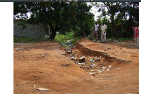
Additional channel on underground pipe culvert arranged by community, Coleman Ave.
