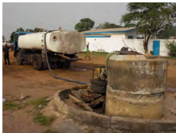
Figure 2.5-6 Groundwater Well at Airfield
