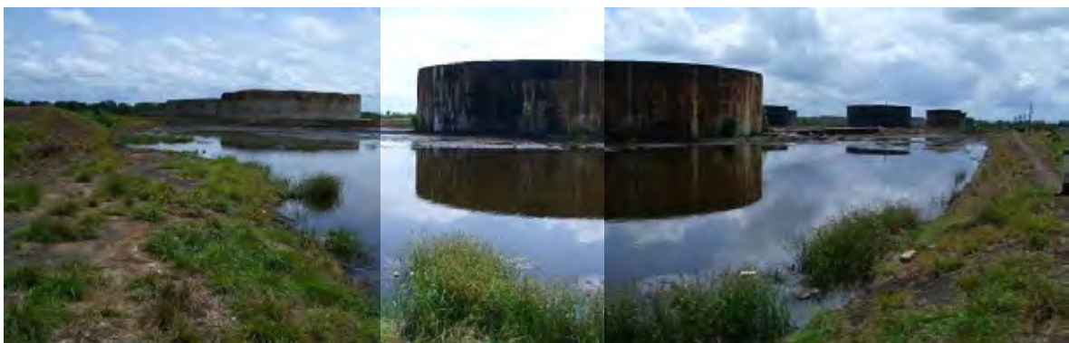
Figure 2.5-37 Present State of Old Refinery Facility
