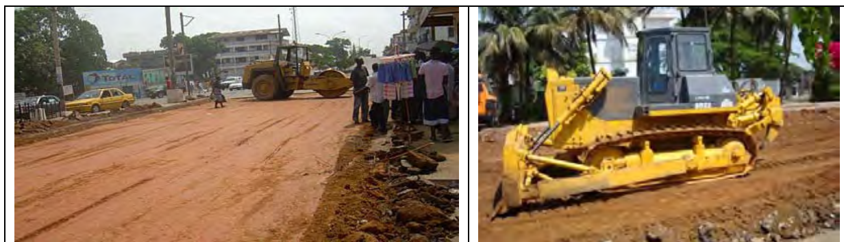
Figure 2.4-6 Rehabilitation Work on Broad Street in CBD Monrovia (March 2009)
