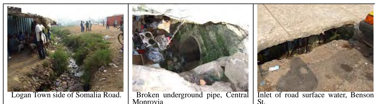
Figure 2.13 Existing Condition of Drainage System
