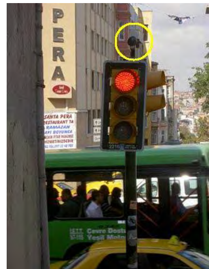
Figure 6.1.1 Camera Detector on Top of Signal Lantern
