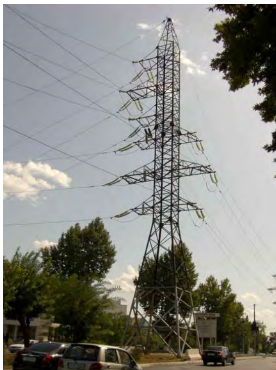
Figure 1-2-7 Example of typically used T-junction Tower
