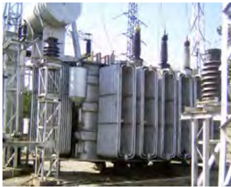
Figure 2-1-5 Step-up transformer
