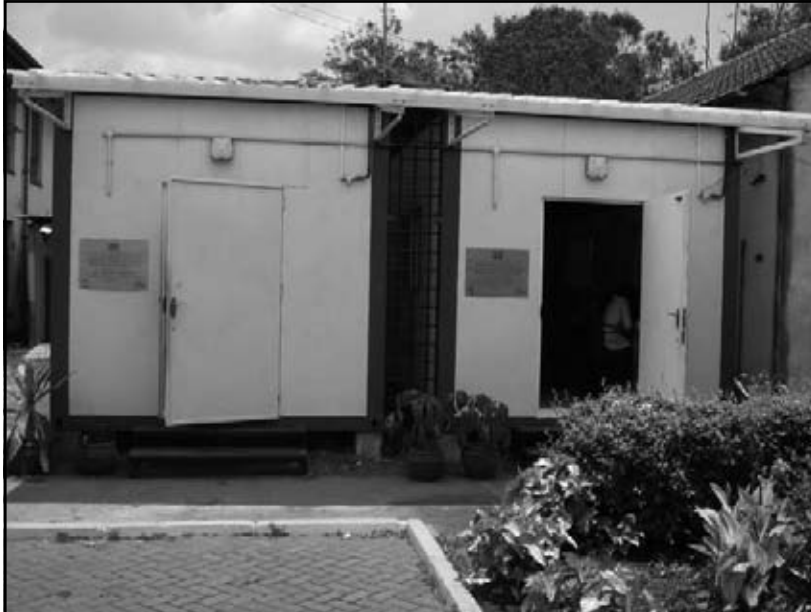
Front View of SPEAK Project Office
