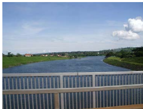
Kiira Power Station (200 MW=4 Units x 50 MW)
