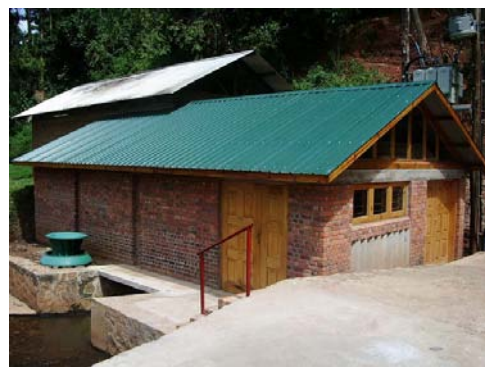
New Powerhouse completed in Feb. 2009
