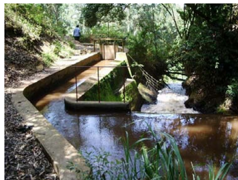
Intake of Power Station
