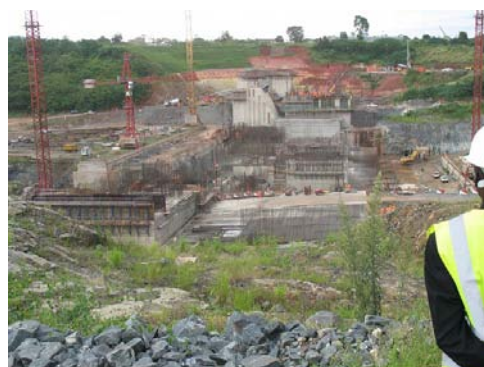
Construction of Powerhouse (5 Units x 50 MW, Photo by MEMD)
