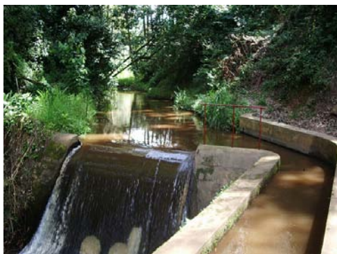
Intake Weir of Power Station
