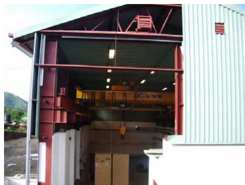
Powerhouse (13 MW, 2 Units x 6.5 MW)
