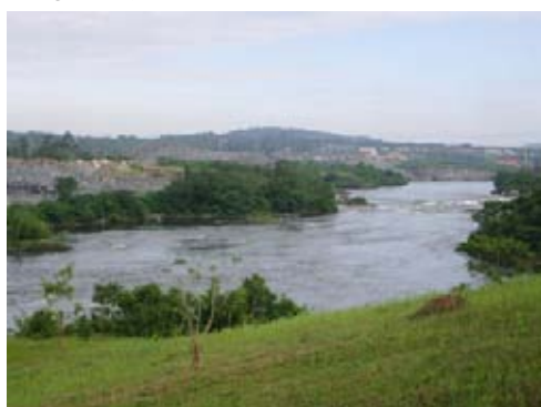
Construction Works on Left Bank, Planned Completion in 2011
