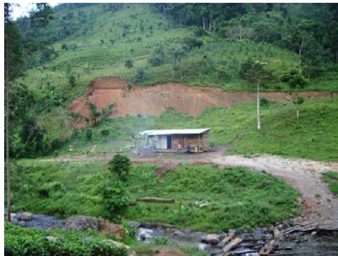
Construction Site of Waterway and Powerhouse
