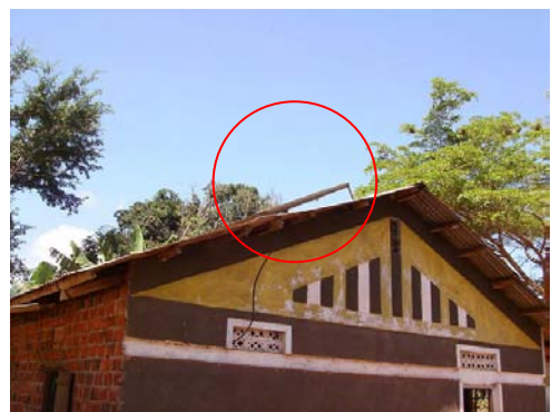
2 Sets of PV Modules of 120 Wp
