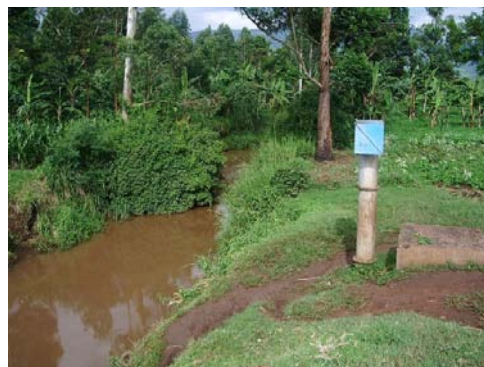
Automatic Water Level Gauging Station
