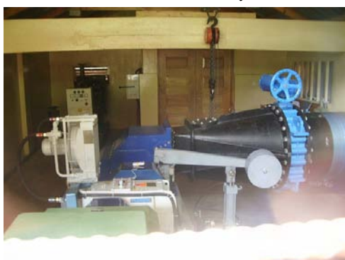
Head 50 m, Discharge 1 to 1.5 m 3 /sec, 300 kW
