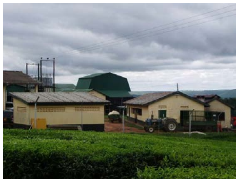
Biomass Gasification Power Plant (205 kW)
