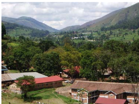
Kisizi Hospital established in 1950s
