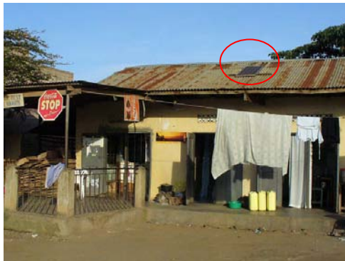
PV Module for Battery Charging
