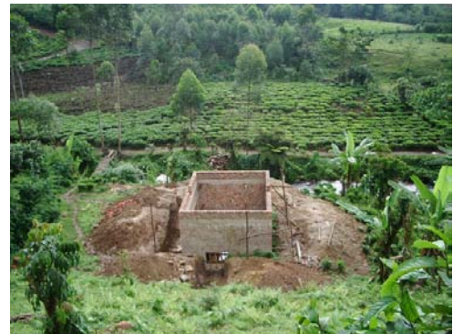
Powerhouse under Construction (Head 40 m, 60 kW)
