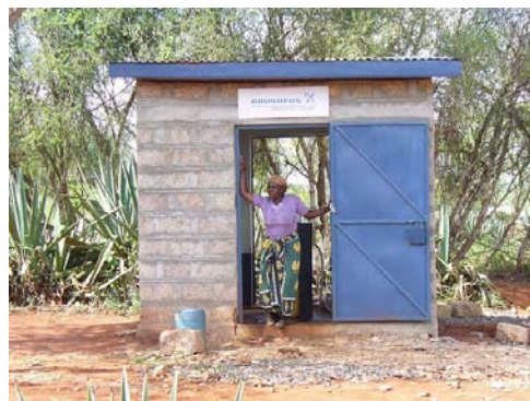
Water Supply House
