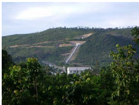
Steel Pipe Lines and Powerhouse
