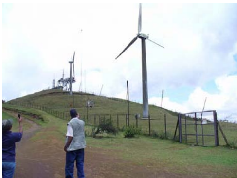
Wind Power Turbines (200 kW & 150 kW)
