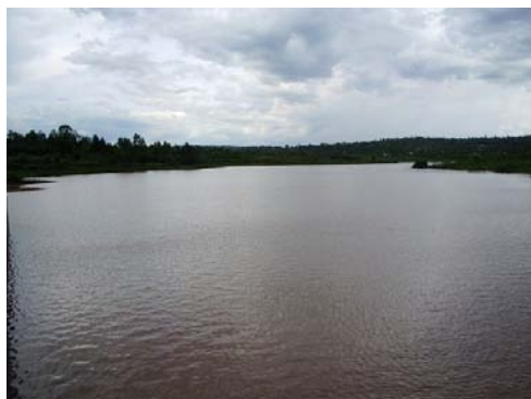
Regulating Pond at Intake Weir in Sondu River
