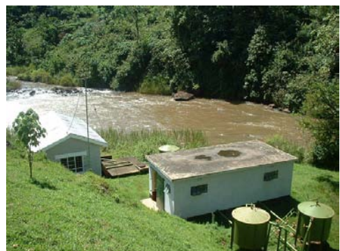
Powerhouse (Left) and Pump house (Right)
