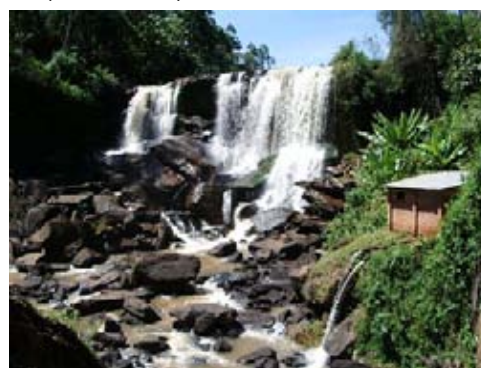
Waterfall and Hydropower Station
