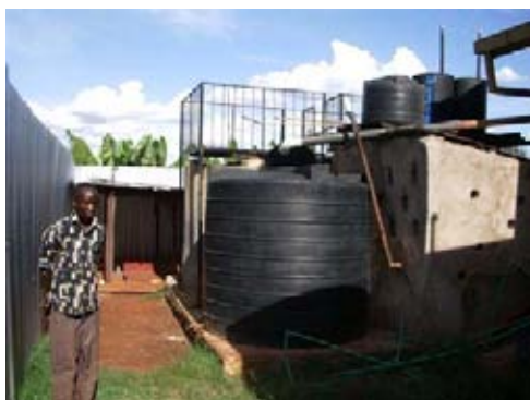
Hydrolysis Tank with Banana Trunks
