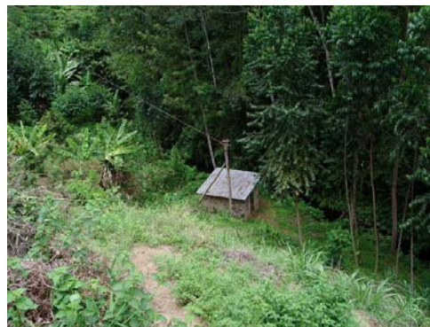
Power Station about 50m below the Intake
