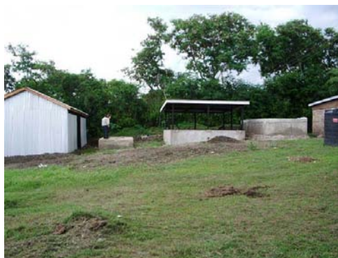
Biogas Facility under Construction supported by UNIDO & KIRDI
