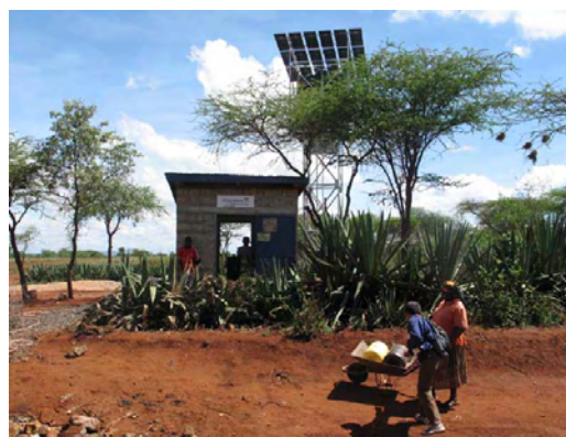
Tube-well by PV pumping operated by Grundfos
