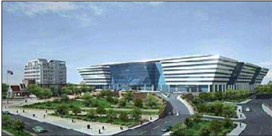
Picture 1: Entrance of the Complex
