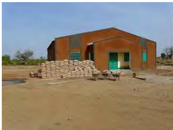
CSPS 建物外観 (Manga)
