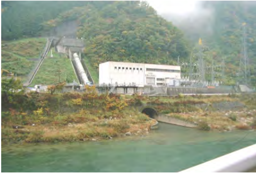
Photograph 51-3 Ground Surface Type Powerhouse and Outlet
