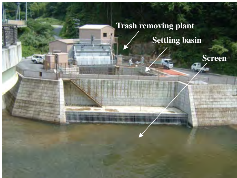
Photograph 43-1 Intake of Run-of-River Type Hydropower Station
