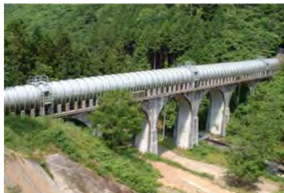
Photograph 45-4 Steel Pipe Type Aqueduct
