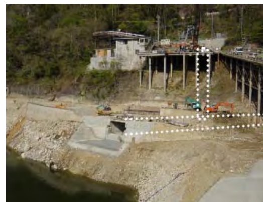
Photograph 43-3 Construction of Reservoir Type Intake
