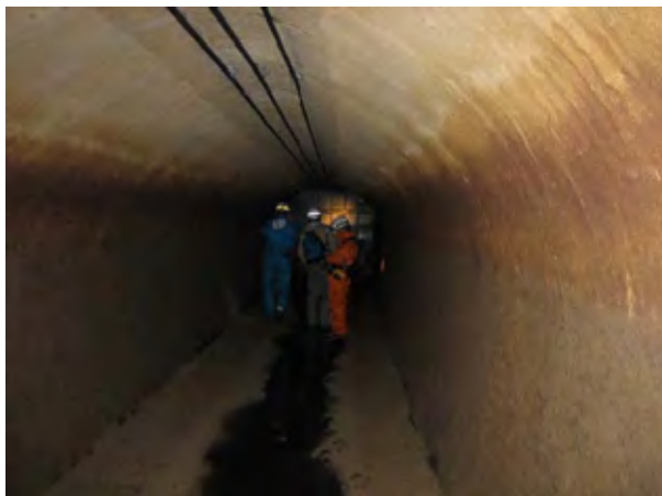
Photograph 45-1 Horseshoe Shaped Non-Pressure Tunnel
