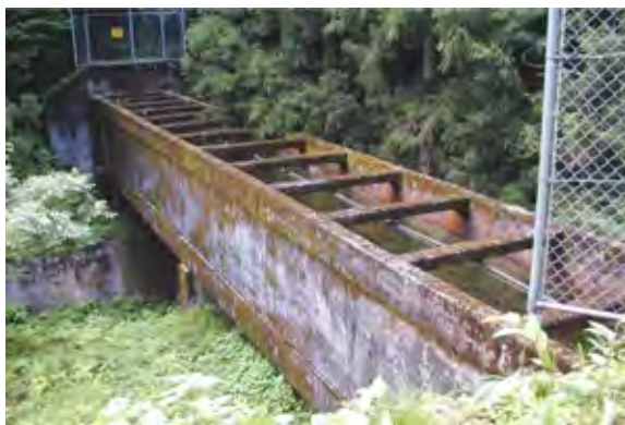
Photograph 45-3 Concrete Type Aqueduct
