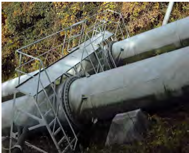
Photograph 48-4 Expansion Joint and Scaffold for Inspection of it
