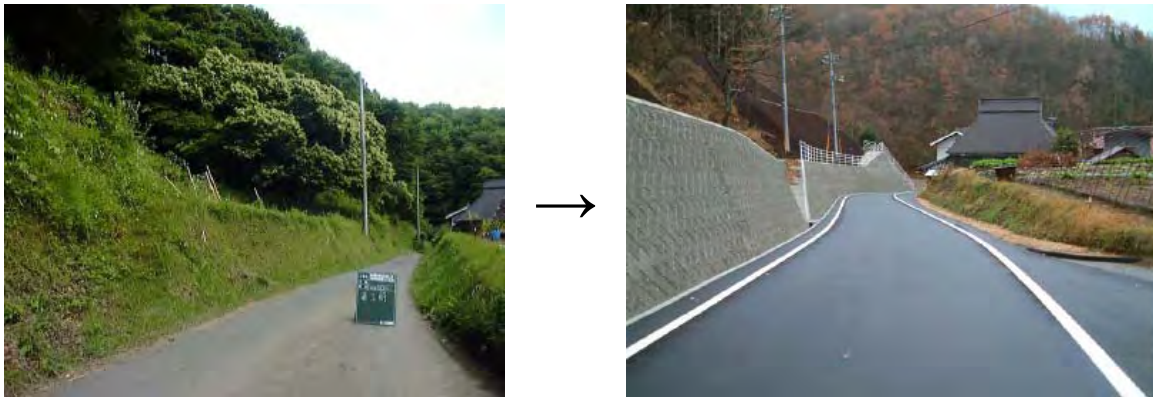
Photograph 52-2 Road for Construction and Maintenance (opened to the public)
