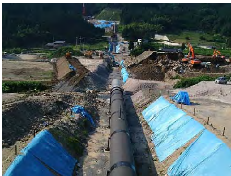
Photograph 45-5 Inverted Siphon under Construction
