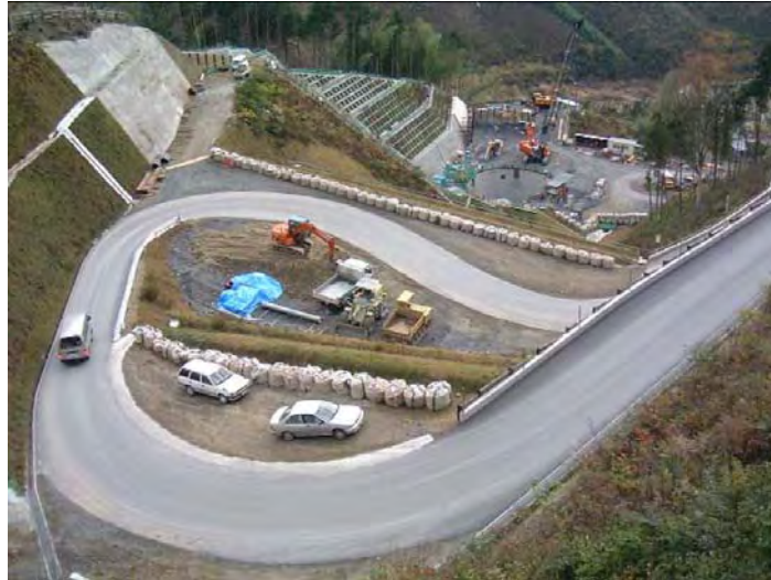
Photograph 52-1 Temporary Road for Construction
