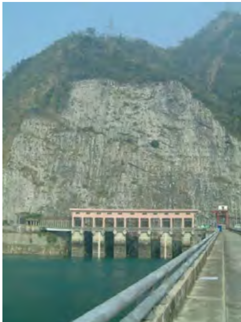
Photograph 43-1 Intake of Run-of-River Type Hydropower Station
