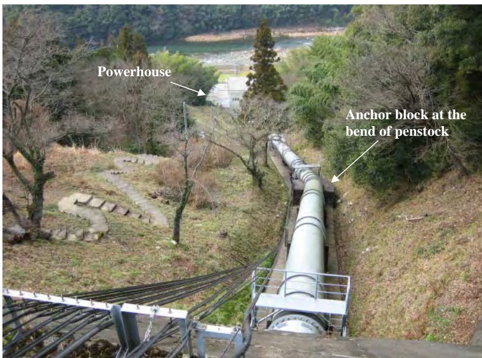
Photograph 48-2 Penstock View from Head Tank
