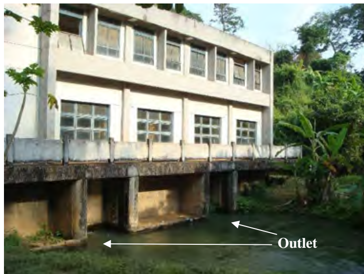
Photograph 49-1 Powerhouse and Outlet of O'Chum 2 Hydropower Station
