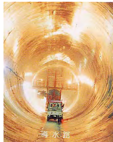
Photograph 45-2 Circular Shaped Pressure Tunnel
