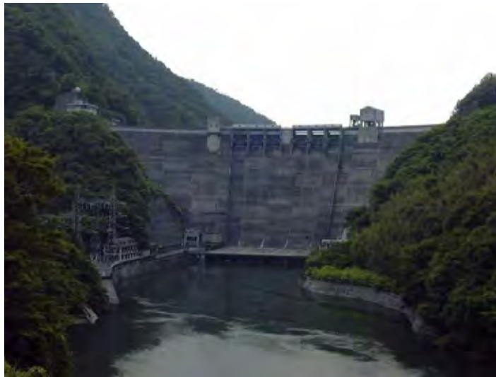
Photograph 39-2 Spillway with Gate (Semi-Hydraulic-Jump Type)
