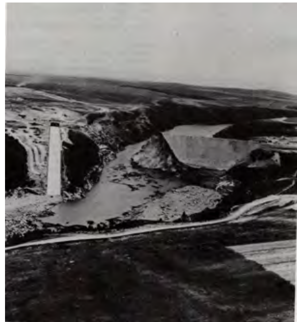
Photograph 15-1 Overflow of Dam (Teton Dam Case in the USA)
