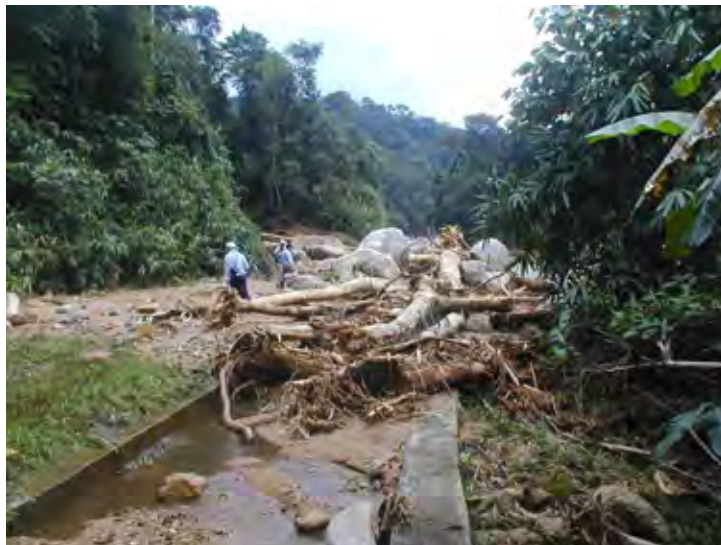
Photograph 17-1 Inflow of Sand or Silt Particles into a Waterway
