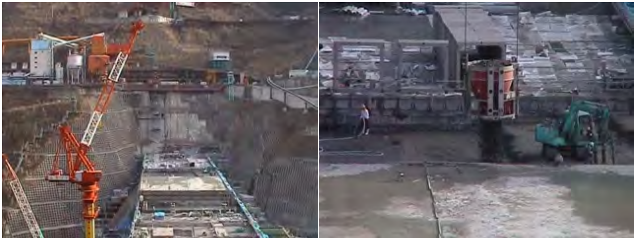
Photograph 27-1 Placing of Dam Concrete
