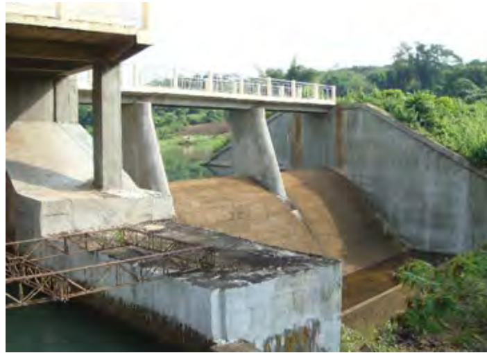
Photograph 39-1 Downstream of O'Chum 2 Dam Spillway with No Gate (Hydraulic-Jump Type)
