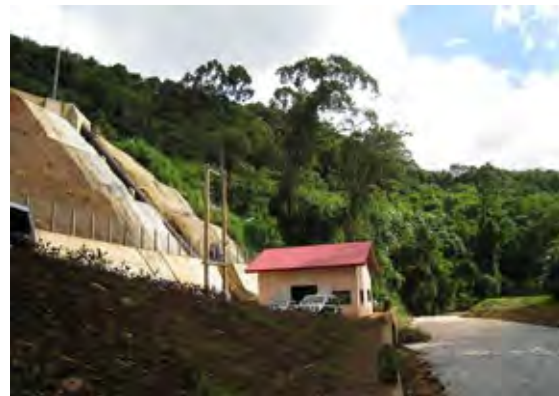
Photo 5.4-4 Powerhouse (O'Romis Hydropower Project)
