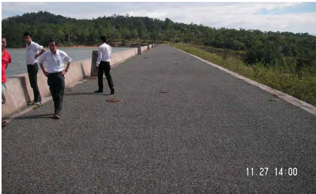
Photo 5.3-2 Dam Crest, Kirirom 1 Hydropower Station (2/2)
