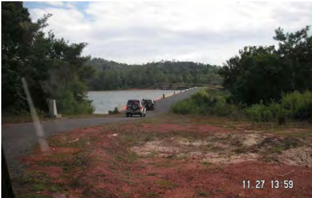
Photo 5.3-1 Dam Crest , Kirirom 1 Hydropower Station (1/2)
