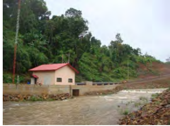
Photo 5.4-2 Powerhouse (O'Moleng Hydropower Project)
