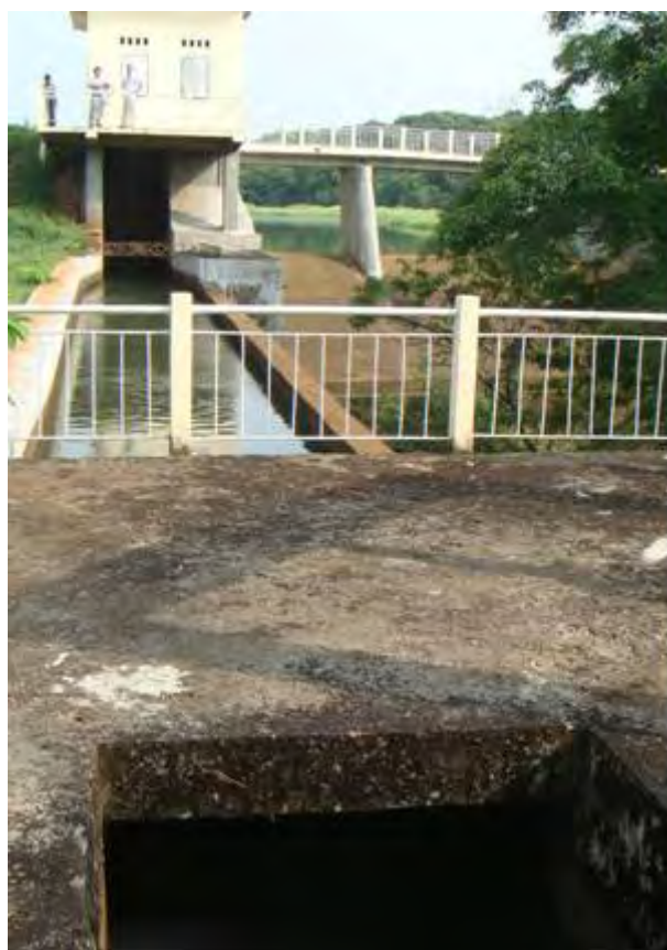
Photo 5.2-3 Intake and Spillway at O'Chum 2 Dam (from the sand basin)
