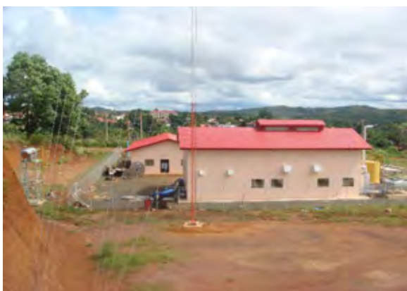
Photo 5.4-5 Diesel Power Station (this side) and Administration Building (left side)
