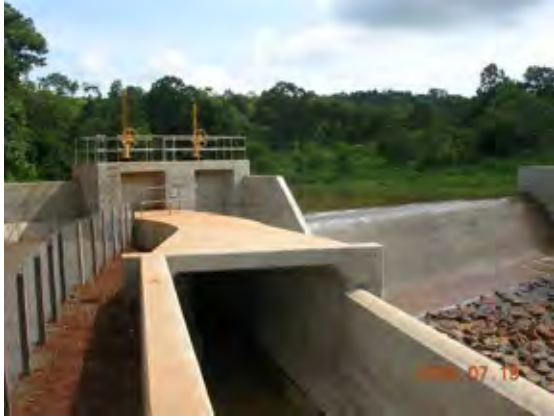
Photo 5.4-1 Intake Weir and Settling Basin (O'Moleng Hydropower Project)
