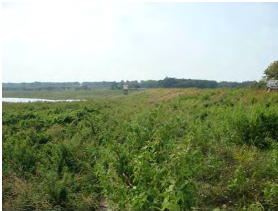
Photo 5.2-1 Upstream Face of O'Chum 1 Dam and Intake Tower (from the right bank)
