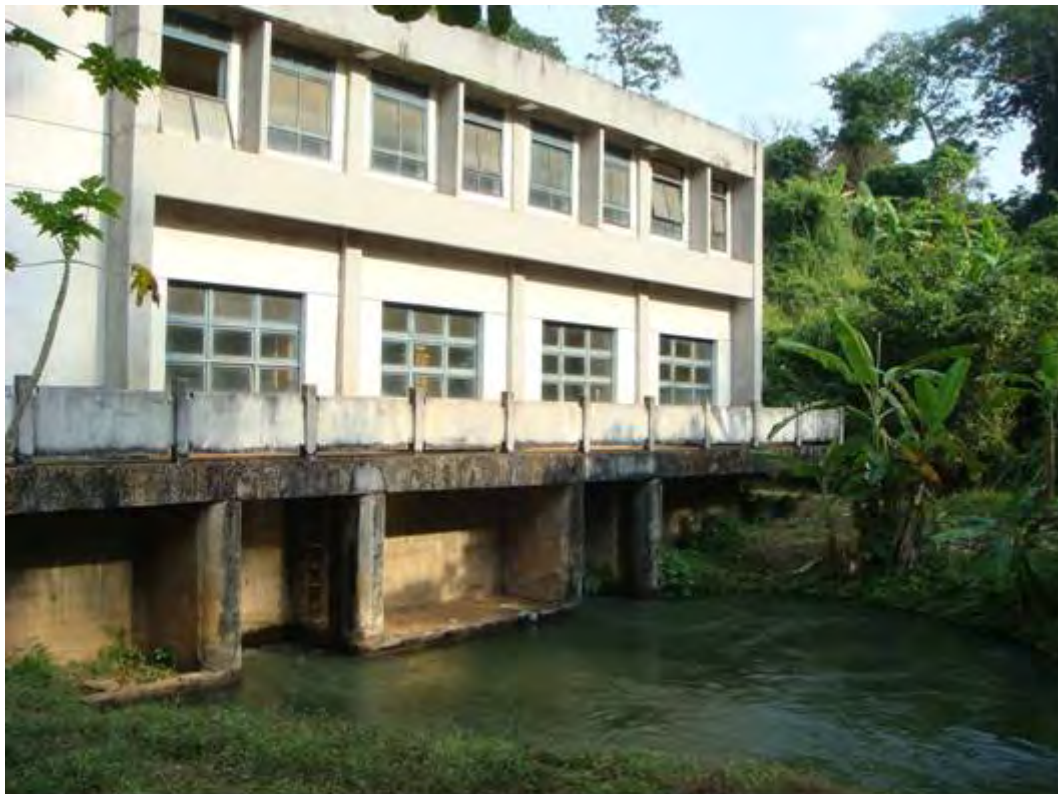
Photo 5.2-9 Powerhouse and Outlet of O’chum 2 Hydropower Station
