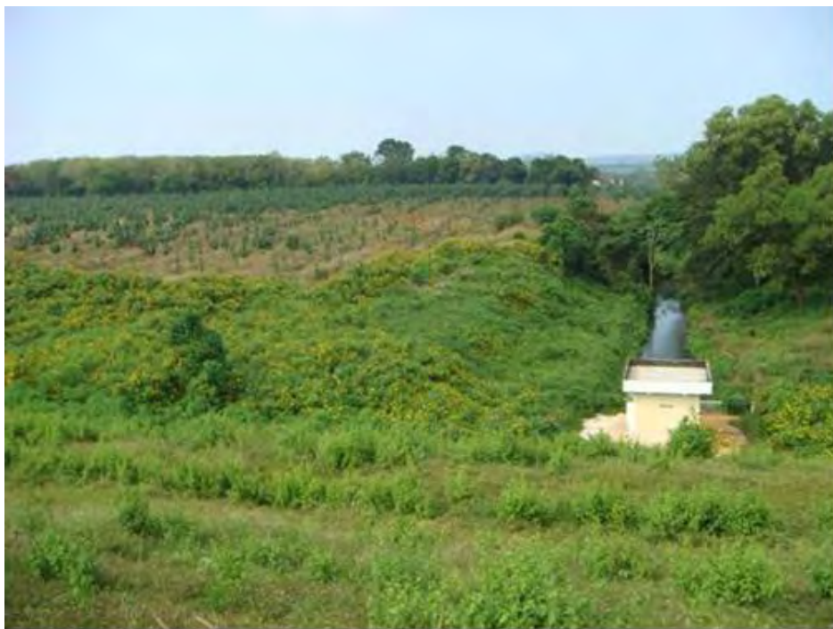
Photo 5.2-2 Downstream Face of O'Chum 1 Dam, Dissipating Valve House and Open Channel to O'Chum 2 Dam
