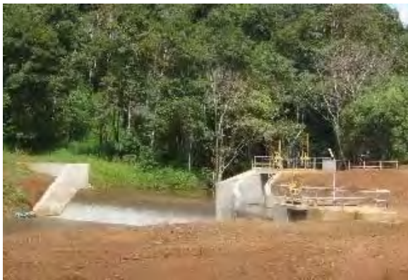
Photo 5.4-3 Intake Weir and Settling Basin (O'Romis Hydropower Project)
