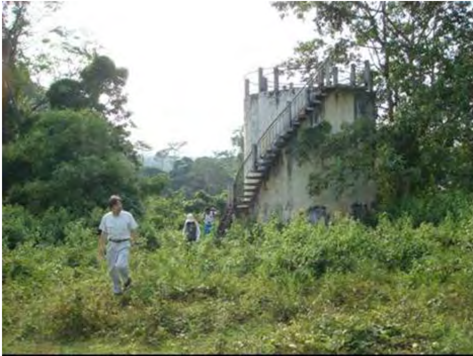
Photo 5.2-4 Surge Tank of O'chum 2 Hydropower Station
