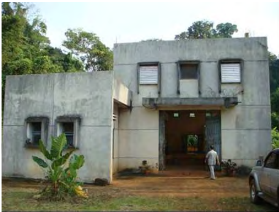
Photo 5.2-5 Powerhouse of O'chum 2 Hydropower Station
