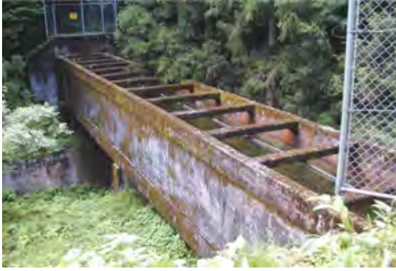
Photograph 45-3 Concrete Type Aqueduct
