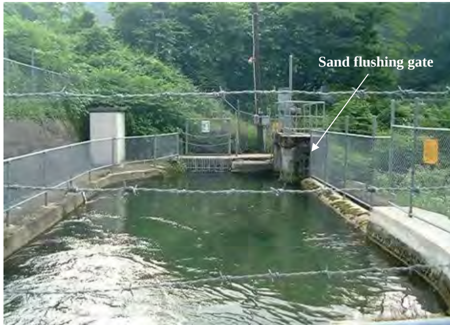
Photograph 44-2 Settling Basin of the Other Station
