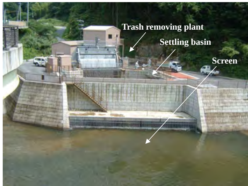
Photograph 43-1 Intake of Run-of-River Type Hydropower Station
