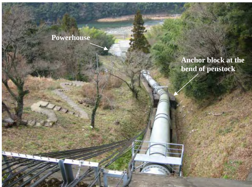
Photograph 48-2 Penstock View from Head Tank
