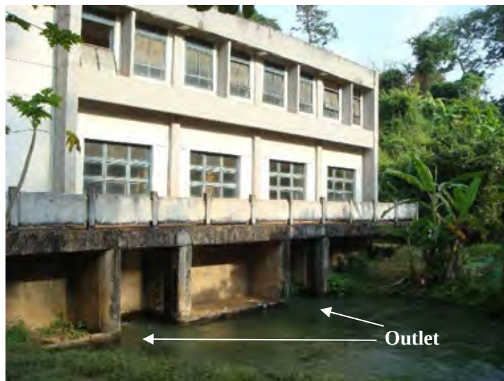
Photograph 49-1 Powerhouse and Outlet of O'Chum 2 Hydropower Station
