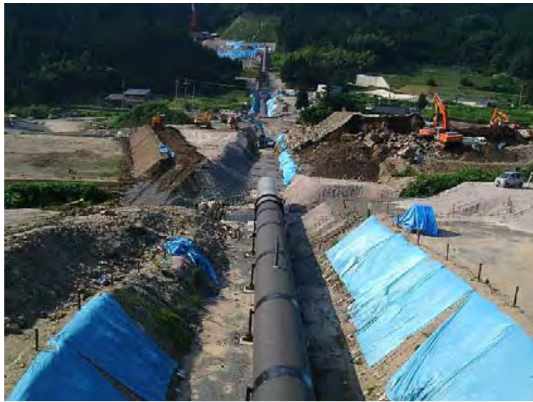
Photograph 45-5 Inverted Siphon under Construction
