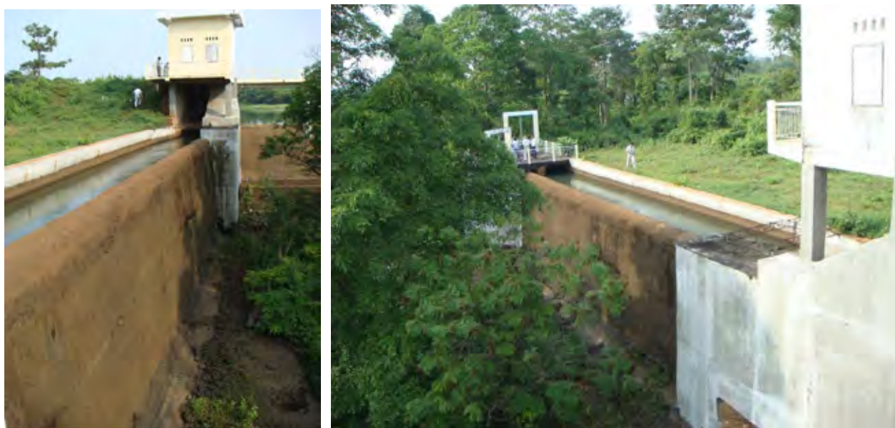
Photograph 44-1 Settling Basin of the O'Chum 2 Hydropower Station
