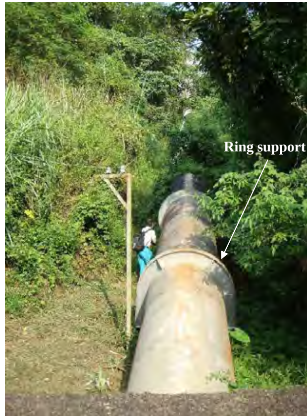
Photograph 48-1 Penstock of O'Chum 2 Hydropower Station
