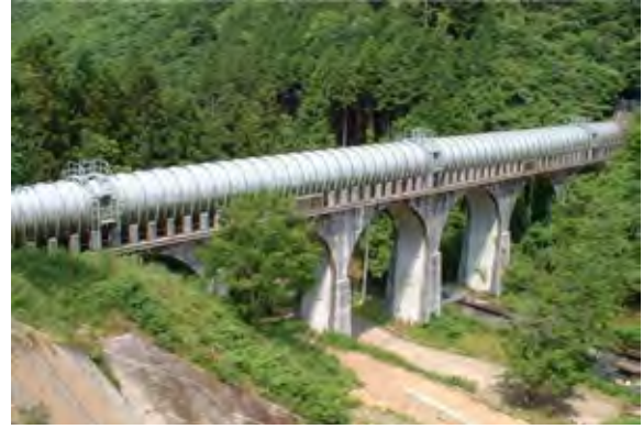
Photograph 45-4 Steel Pipe Type Aqueduct
