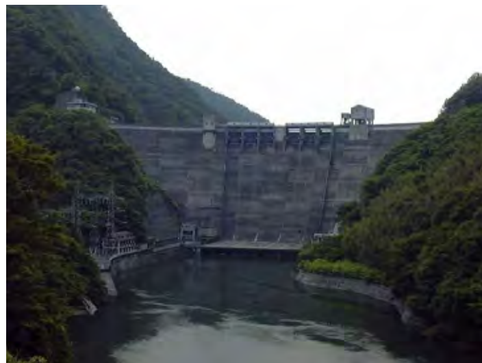
Photograph 39-2 Spillway with Gate (Semi-Hydraulic-Jump Type)
