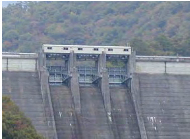
Photograph 40-1 Spillway Gate (Radial Gate) and Hoist
