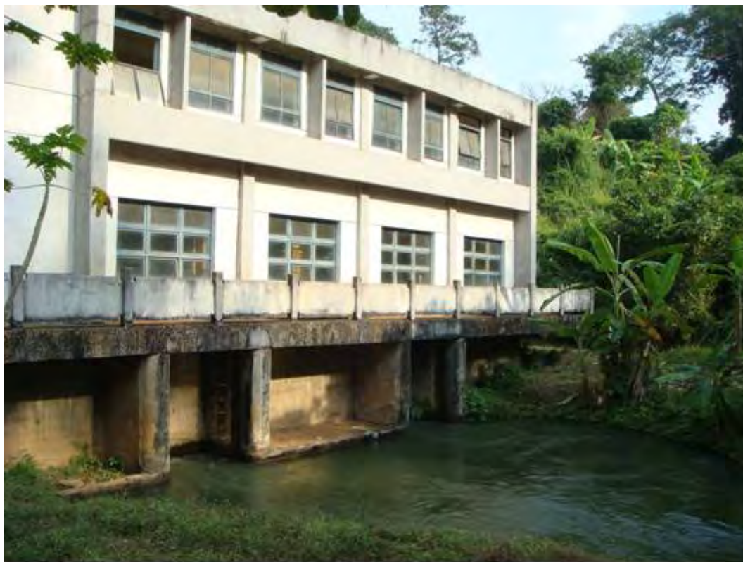
Photo 5.2-9 O'chum 2 発電所建屋と放水口
