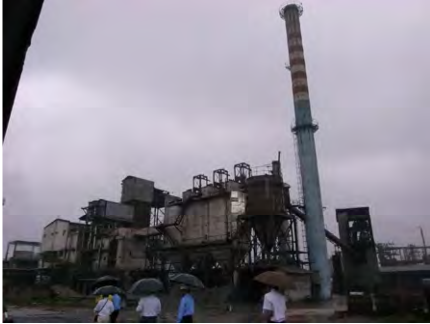
Picture 7-A Waste Heat Recovery System
