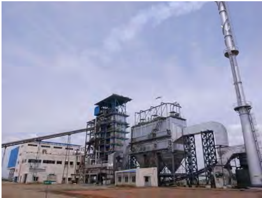
Picture 7-D Biomass Power Generation System
