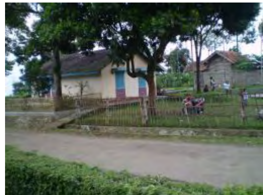
Proposed site for water treatment plant
