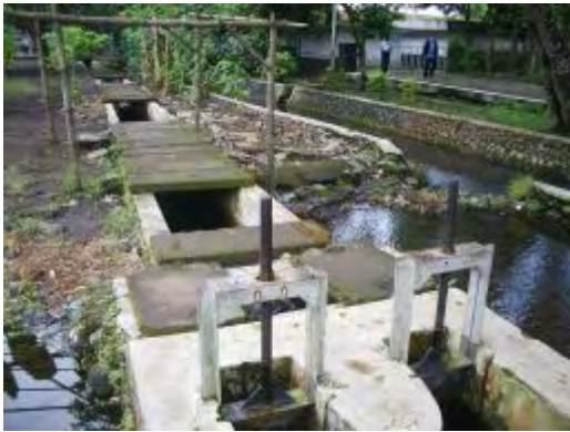
Existing Intake for Irrigation
