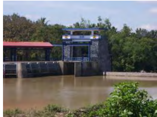
Existing irrigation weir on Garang River
