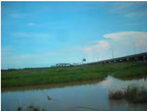
Bandara Juanda (Beginning project)
