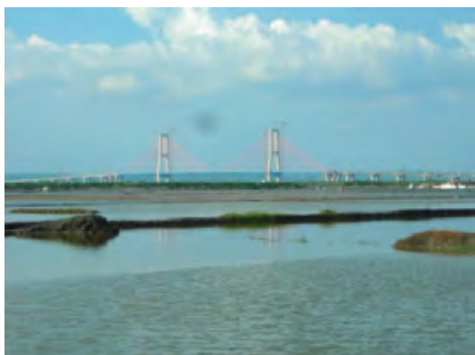
Newly opened Suramad Bridge
