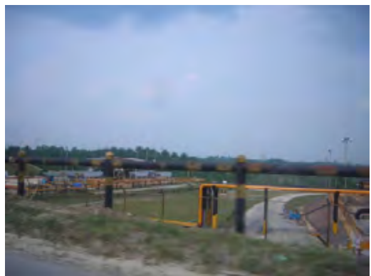
Chevron oil field along ordinary road
