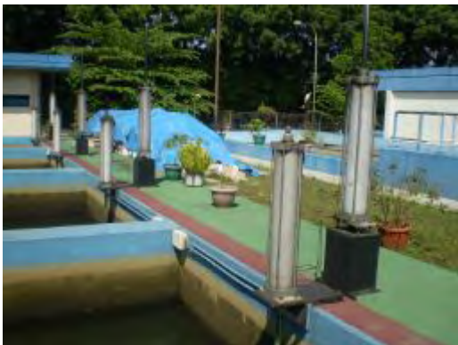
Existing water treatment plant
