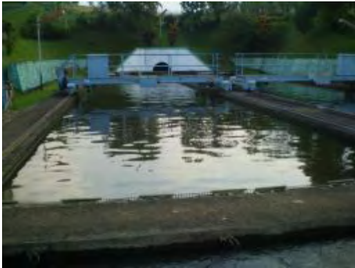
Existing sedimentation basin
