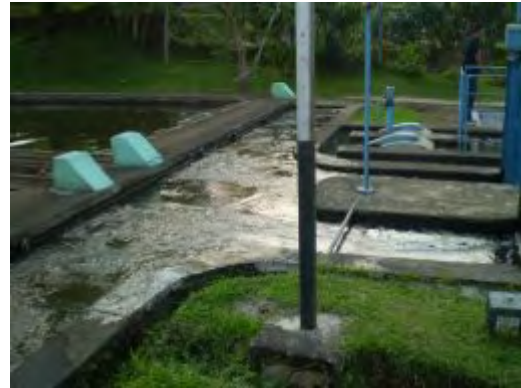
Existing raw water canal
