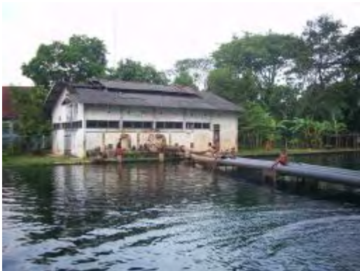
Existing Intake for Irrigation (Pump station)
