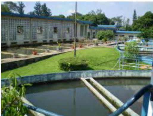
Existing water treatment plant
