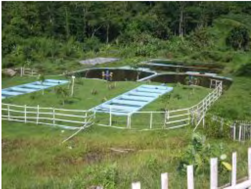
Existing west water treatment plant
