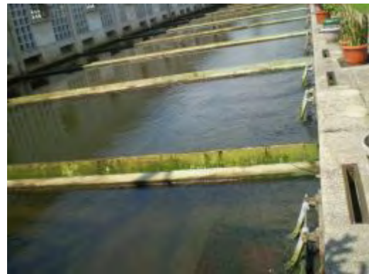
Existing water treatment plant
