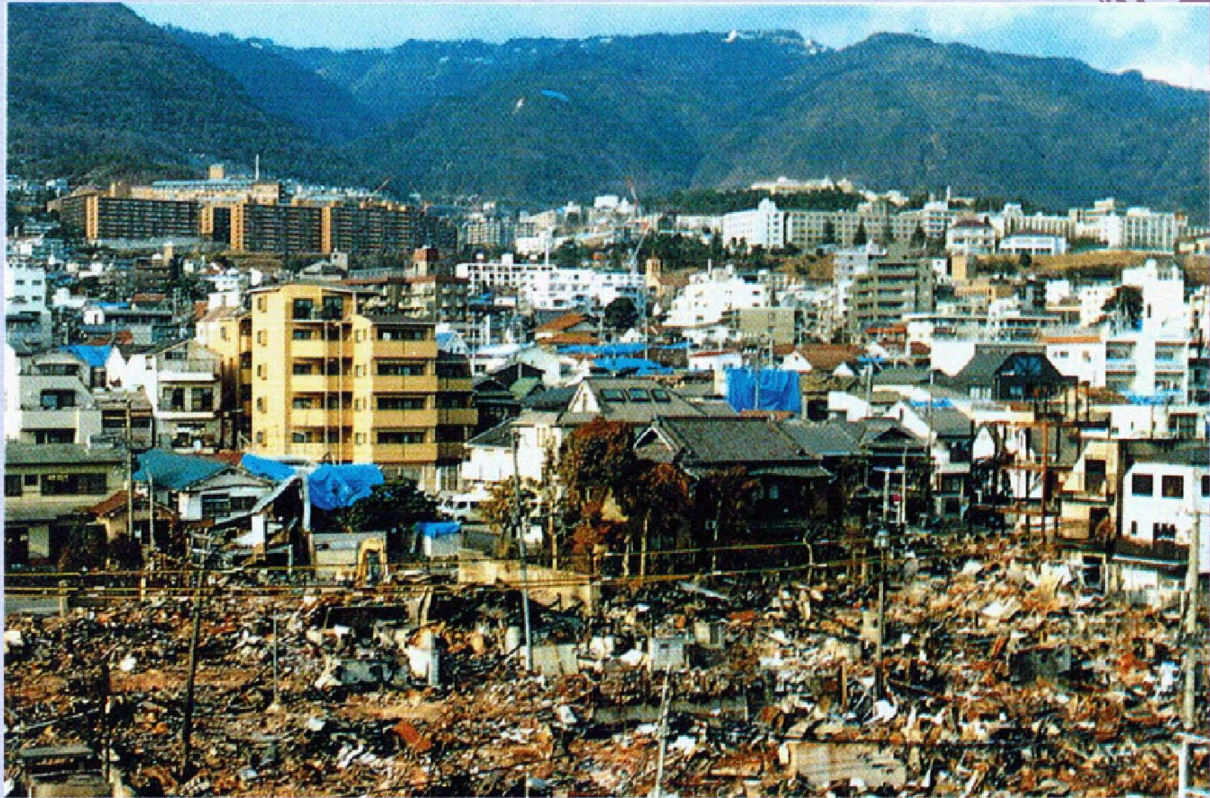
Damages near JR Rokko Station looking at Kobe University
