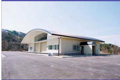
Tajima Regional Emergency Management Base
