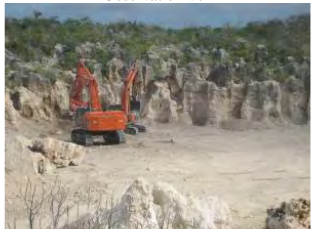
The uneven ground surface is being leveled.
