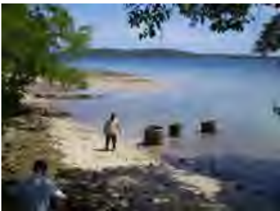
Spring water intake point (Freshwater wells up inside Hume pipes)
