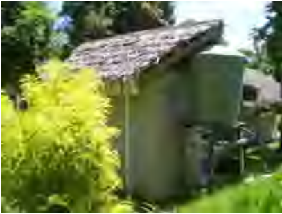
Surface water storage tank for toilet use (Emuwa Village in the north)
