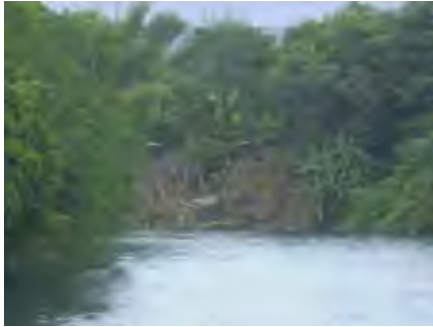
Bank collapse upstream of Sarakata River
