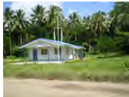
Police station rainwater storage tank for drinking (Ditto)
