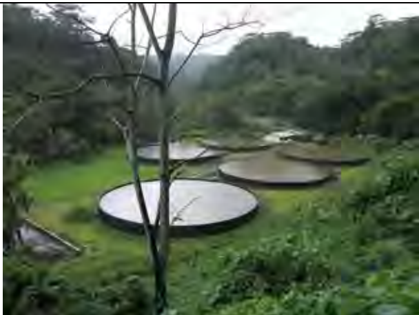
Main water treatment plant in Capital City Apia (slow filtration plant in ALAOA). Turbidity of water become high by torrential rainfall, and filter is clogged with mud.
