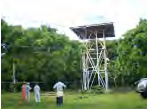
Existing elevated tank voltage distribution
