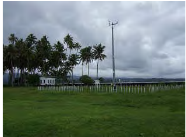
Yard of Meteorological observation station in Samoa (provided by Japan) is inundated by high tide in a cyclone
