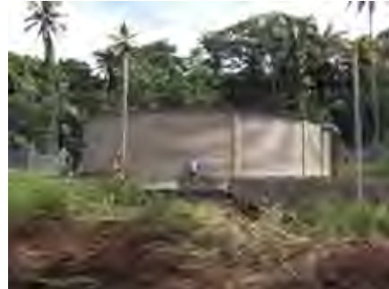
Receiving tank (not in use)
