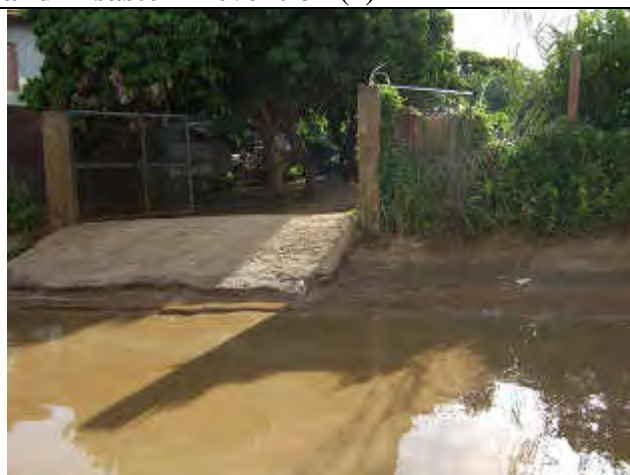
Flood in is usually occurring and embankment is constructed to prevent overflowing of flooding water at 7-star area of Portville, Capital of Vanuatu.
