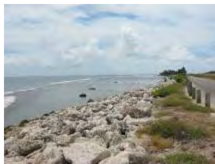
Photo 2-2.2 Area around Airport Runway Landfill
