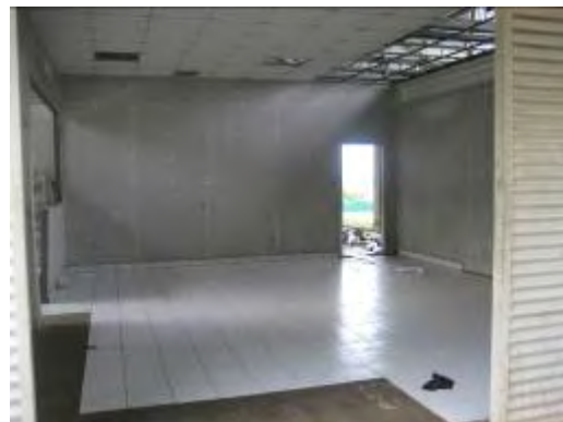
Equipment workshop (unfinished)
