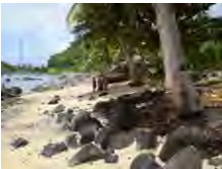
Tree roots exposed by scouring
