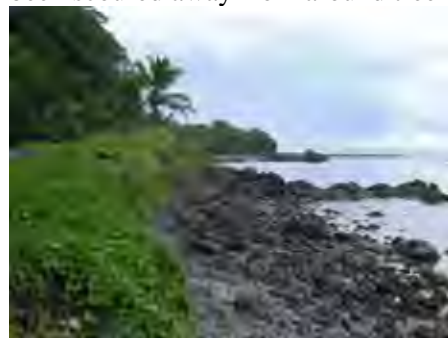
High tide damage encroaching the road
