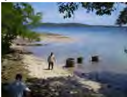
Spring water intake point (Freshwater wells up inside Hume pipes)
