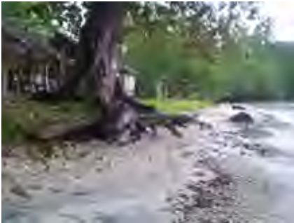
Coastal erosion in the south (Naruruna Village) (Seawater comes up to the market here)
