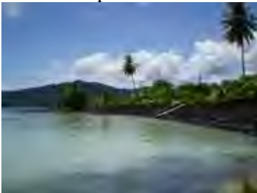
Seawall constructed in the project
