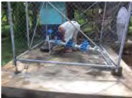
Bore hole installation
