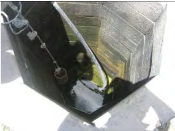
Hand dug well in Kiribati. Sea water intrusion made salinity of groundwater of this well high, and people cannot drink water.
