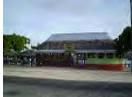
Building for sea bathers in the southeast of the island
