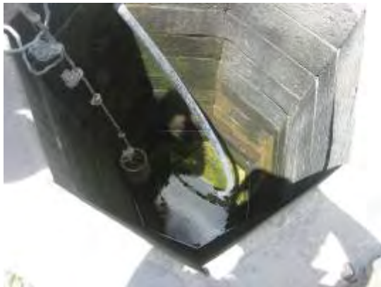
Photo 2-2.3 House well in South Tarawa
