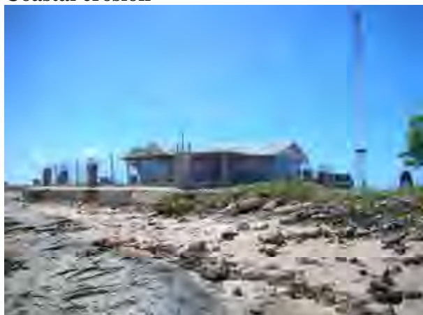
Situation of coastal erosion near Radio station of Kiribati. Part of radio-earth was washed away by erosion.
