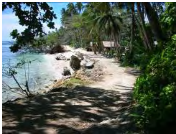
Coastal road in Auki province of Solomon islands. Trunk road is submerged at high water and traffic is interrupted.
