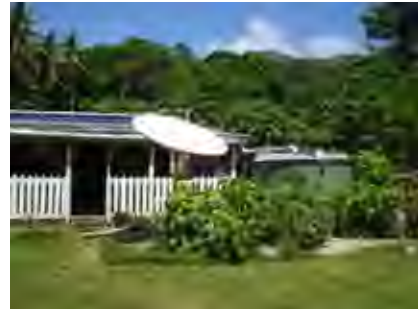
Rainwater storage tank for drinking (Ditto)
