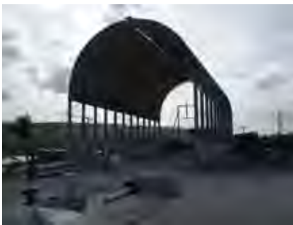
Slipway and tent repair yard
