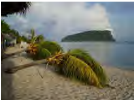
Damage in the southeast of the island
