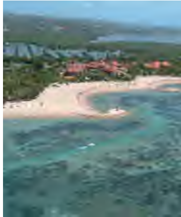
Jetty was constructed against coastal erosion in tourism area (Indonesia, Japanese loan project)
