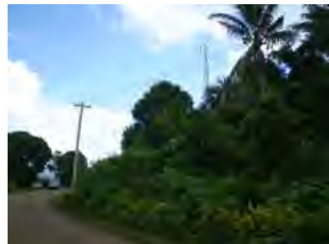
Mobile phone antenna, high lines and other infrastructure have been installed.
