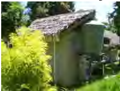
Surface water storage tank for toilet use
