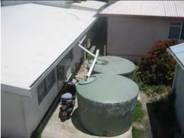
Rainfall tank in Nauru. Many houses have this type of tanks, but it cannot be utilized in dry season.
