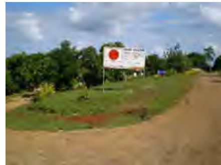
Water supply facilities constructed under Japanese grassroots grant aid
