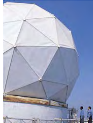
Radar for meteorological observation (Bangladesh, Japanese Grant Aid project)
