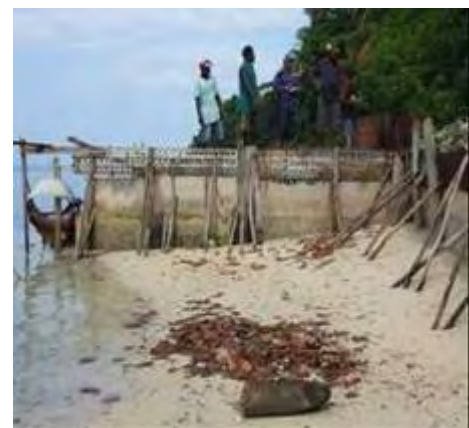
Photo 2-2.5 Coastal Defense Facilities by Residents (Provided by NDC)
