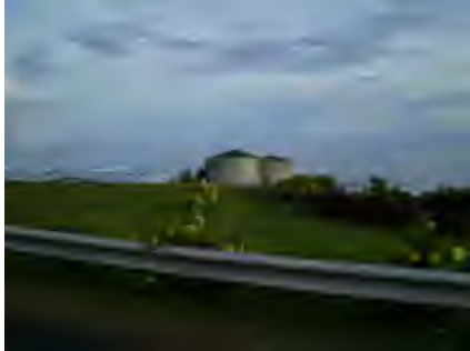
Concrete water storage tanks (Example along coast)
