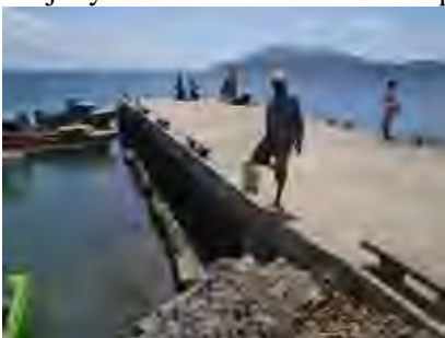
Jetty conditions (Emau Village in the north)
