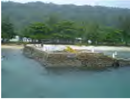
Jetty repaired by the EU
