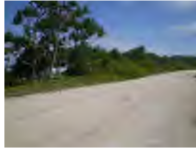
The road is elevated but is sometimes covered by high waves
