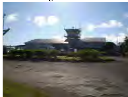
Full view of airport terminal
