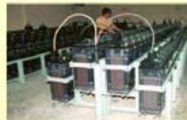
Battery: 600 kWh
