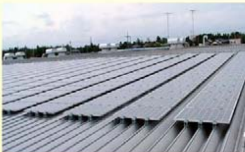
Corrugated Metal Roof
