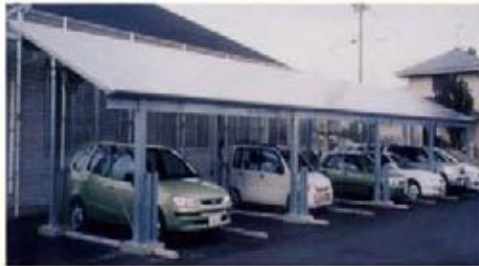
Roof of Carport
