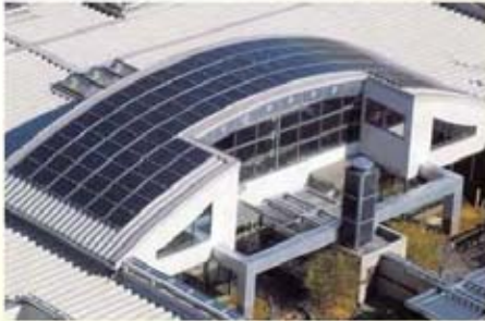
Corrugated Metal Roof
