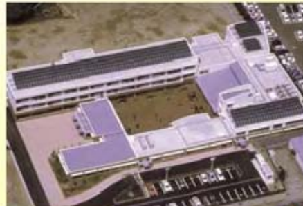
Roof-top of a School
