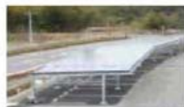
Roof of a parking (30 kW)
