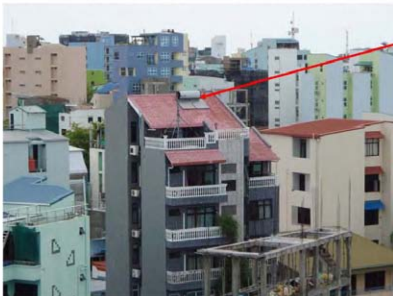
Solar water heater
