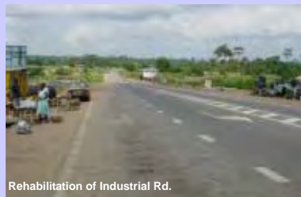
Rehabilitation of Industrial Rd.
