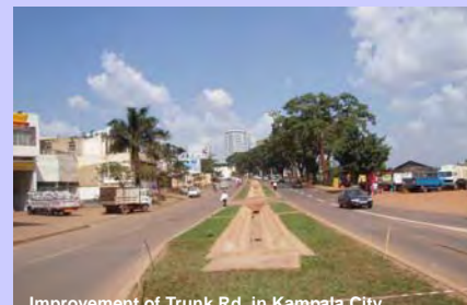
Improvement of Trunk Rd. in Kampala City
