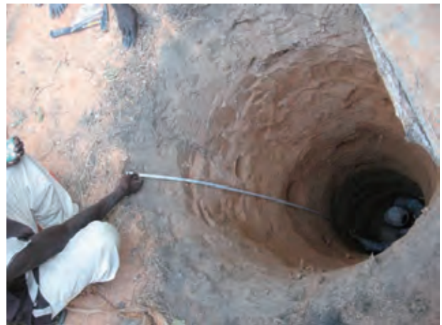
Photo 9 Pit-3 (3m in depth) (Lh7062403)
