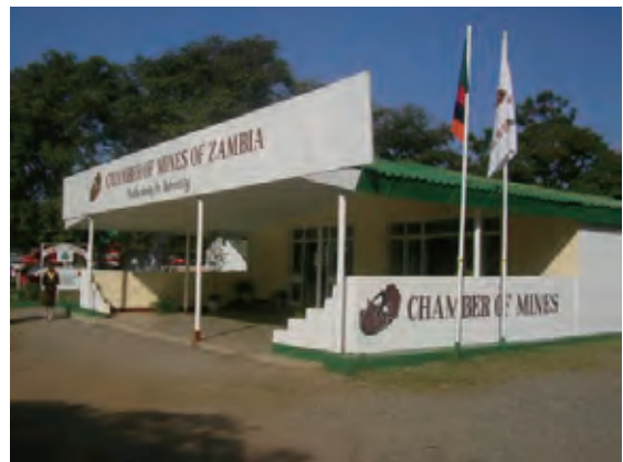
Chamber of Mines pavilion
