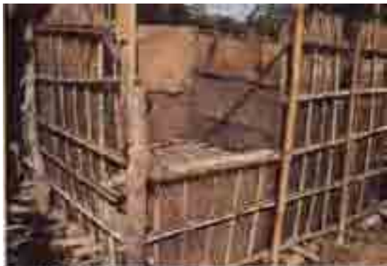
Photo 14: A structure for live treatment constructed with a wooden framework and with walls made from plastic nets (Cambodia) Photo: Kuwait
