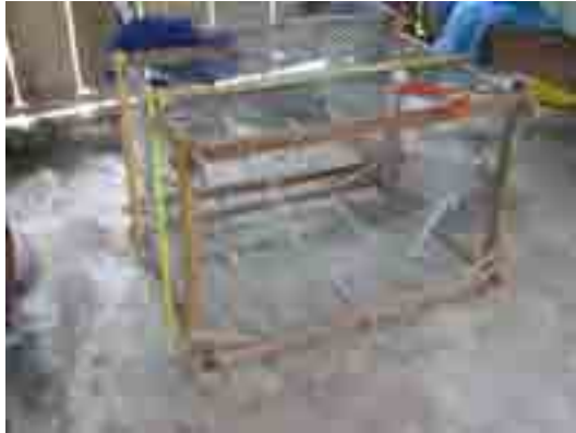
Lumber made frame, fixed with nails
