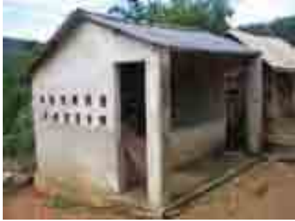
Pigsty with corrugated iron sheet roof, cement floor and wall
