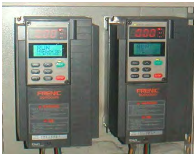
Figure 3.3.2-13 Inverter for Tenter m/c and Dryer Fan
