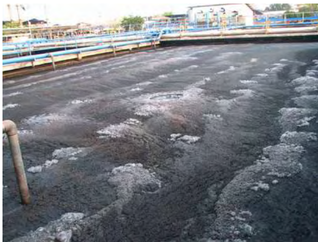
Figure 3.3.2-23 Aeration Tank of Waste Water Treatment of Dyeing Enterprises in Bandung Outskirts
