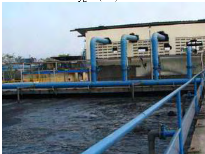
Figure 3.3.2-24 Input Pipe to the Aerating Tank of the Dyeing Enterprise in Bandung Outskirts
