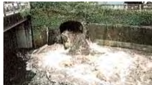
Fig. 5.7 Combined sewer overflow
