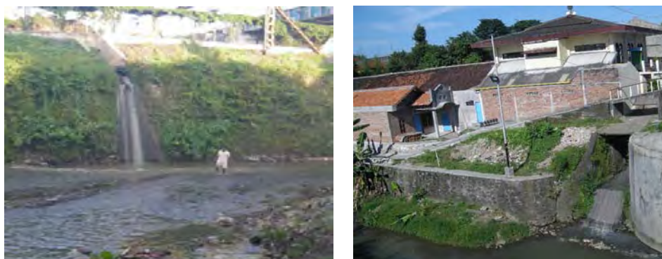
Fig. 8.4 Discharged Wastewater (Drainage in low ground)
