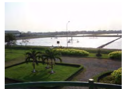
Figure 3.1.17 Binh Hung Hwa WWTP
