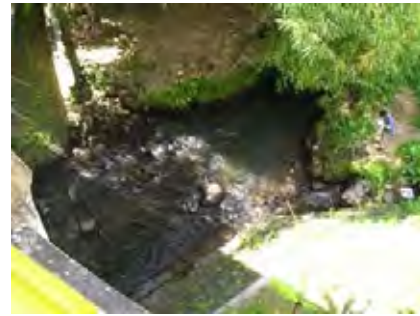
Figure 2.1.14 Drain Pipe in the Upper Part of Code River
