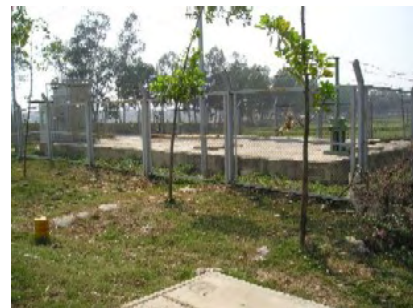
Figure 3.1.5 Relay Pumping Station
