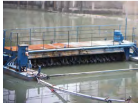
Figure 2.1.7 Surface Aerator
