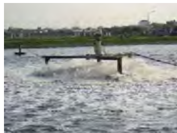
Figure 3.1.24 Surface Aerator
