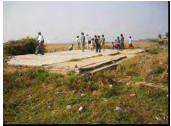
Photo-4: Remain of foundation of old classroom after complete collapse by Nargis. (Bogale No.18-Sat Kyun)
