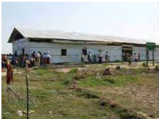
Photo-5: Temporary classroom: Education environment is bad and not safe for cyclone etc. (Labutta No.3-Hlwa Zar )
