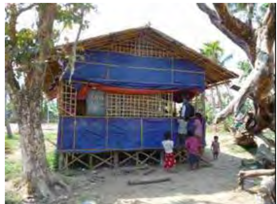
Photo -6: Temporary classroom: shabby wooden or bamboo frame structure covered with plastic sheet. (Labutta No.2-Shwe Gone)
