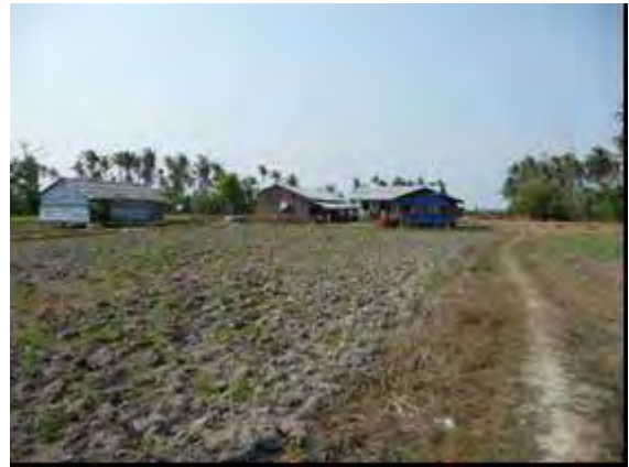
Photo-2: Construction site. Temporary classrooms shall be reconstructed with rigid and safe structure. (Labutta No.17-Tha Pyu Gone)
