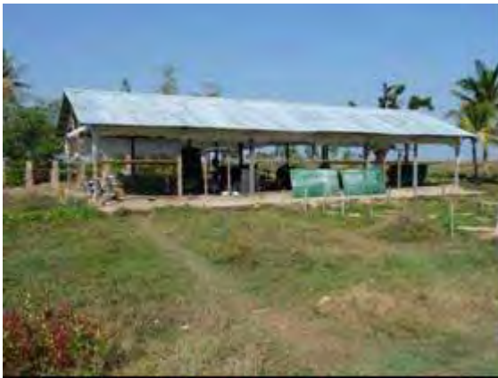
Photo-3: Only roof was repaired temporarily. (Labutta No.4-Zin Pyune Gone)
