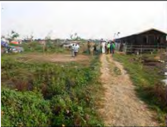
Photo -11: Unpaved road in a village. In rainy season, road condition becomes bad and transportation of construction materials and equipment will get difficult. (Labutta No.15-Ye Kyaw Wa)
