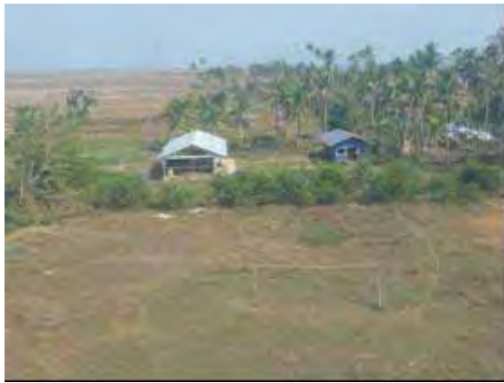
Photo-1: Overview of a flat site. Temporary classroom has only roof sheet without walls. (Labutta No.4-Zin Pyune Gone)
