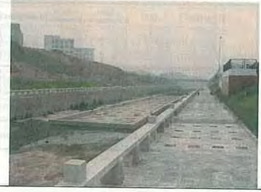
Image of applicable facility in the river with function of STP (Shanghai in China)
