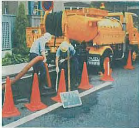
Cleaning of sewer pipes with a high-pressure cleaning truck
