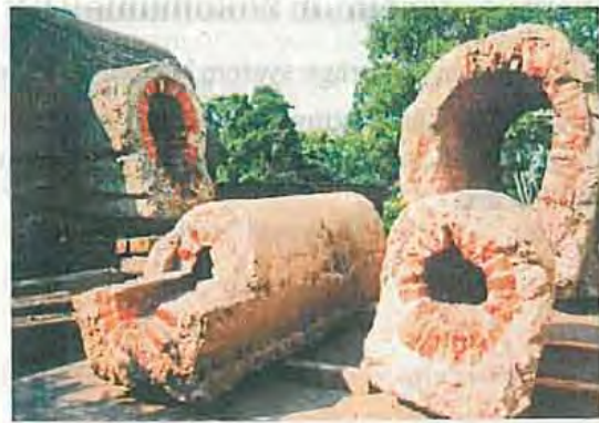
Sewer with an egg-shaped profile
