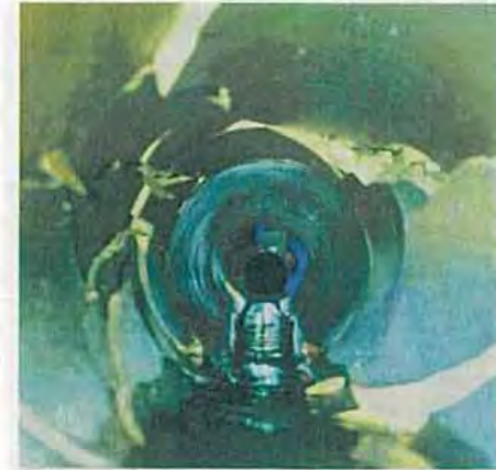
Ruptured pipe (a cause of road subsidence)
