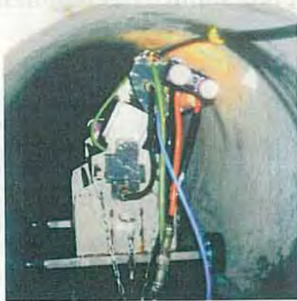
Installation of optical fiber circuits by a robot
