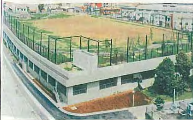
Stormwater tank under the athletic ground
