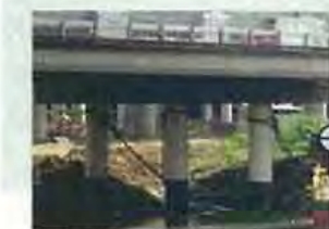
Marcos Highway Outfall
