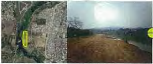
LGU Identified Gawad Kalinga Road Dike Site
