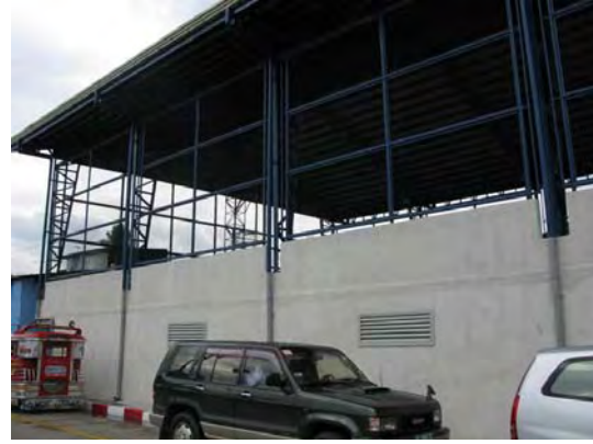
Photo 4.3.4 External view of the completed Capitolyo/Pineda STP.
