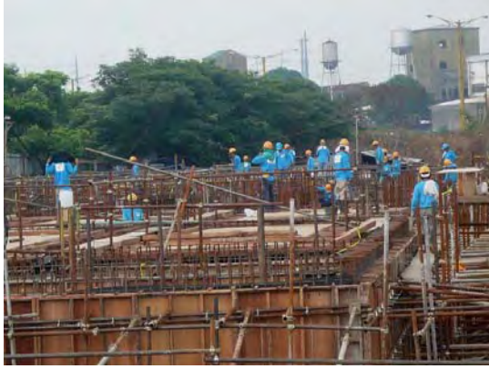
Photo 4.3.3 Construction of the Olandes STP.
