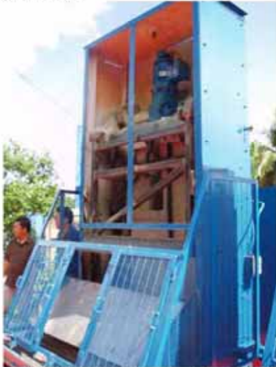
Photo 2.3.3: Flume flow measurement facility
