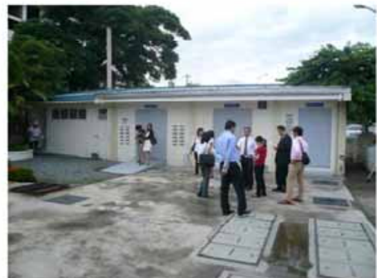
Photo 2.3.6: Centennial STP, an underground STP serving medium-rise residential condominiums. Operated by MWCI
