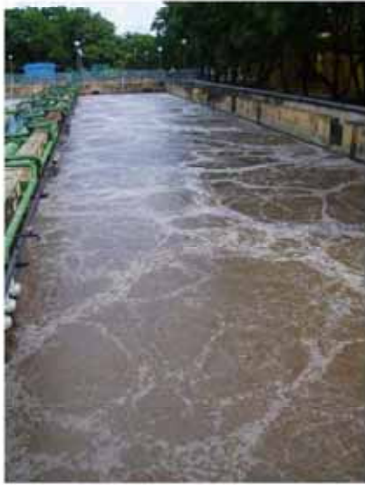
Photo 2.3.1: Sedimentation basin during maintenance
