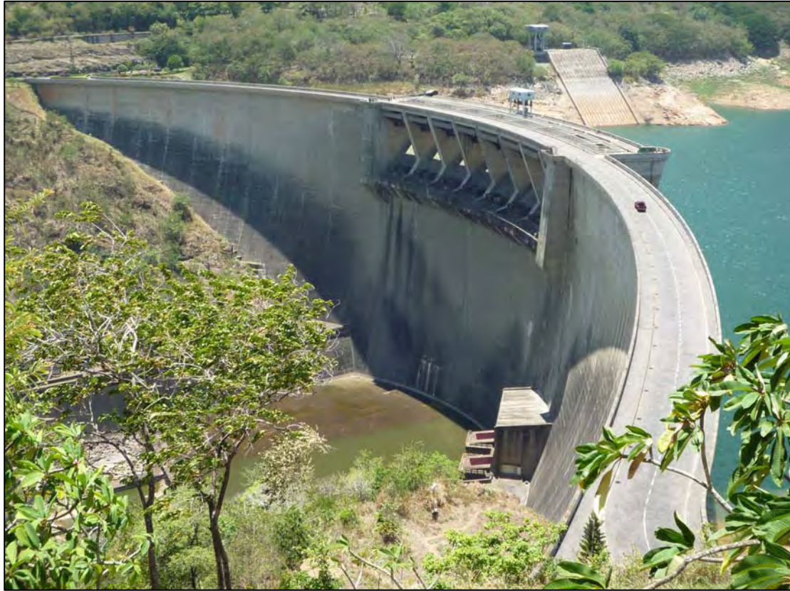
Existing Victoria Dam
