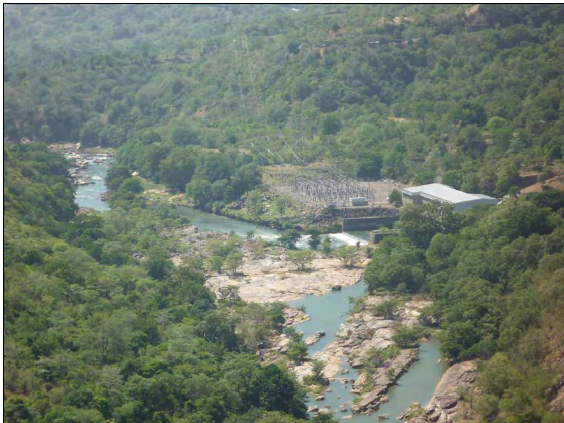
Existing Powerhouse & Switchyard
