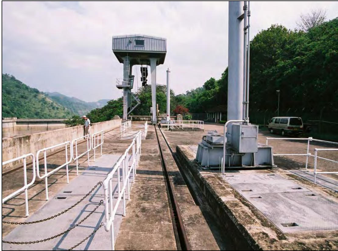
Existing Intake for Expansion
