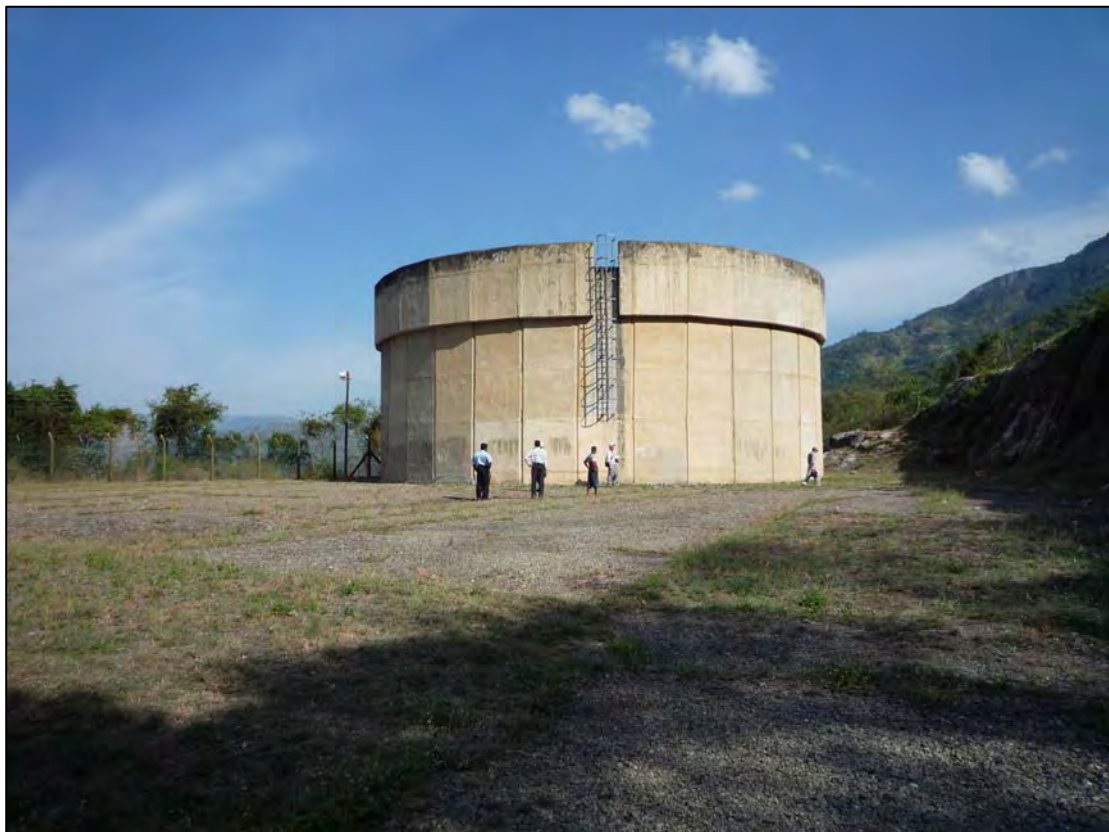
Existing Surge Tank
