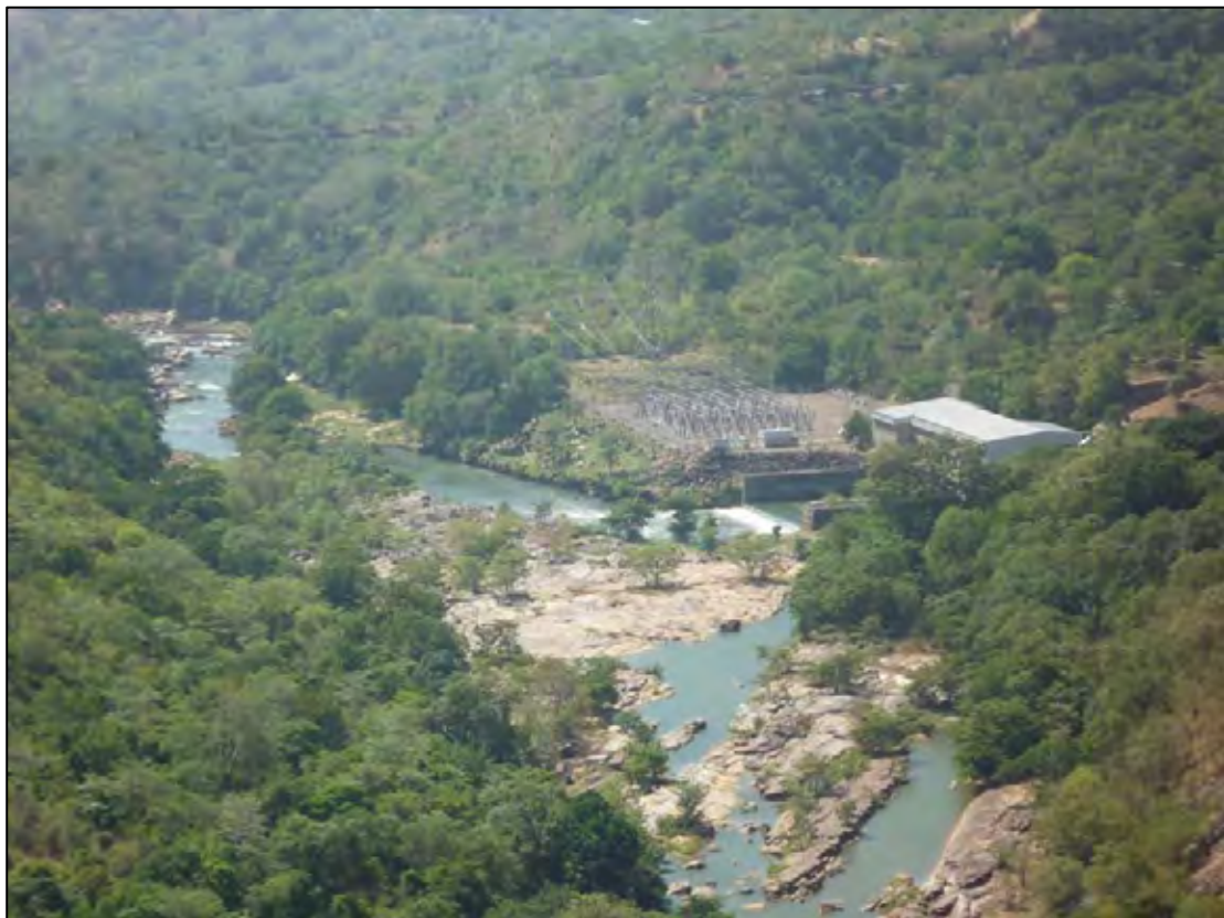
Existing Powerhouse & Switchyard
