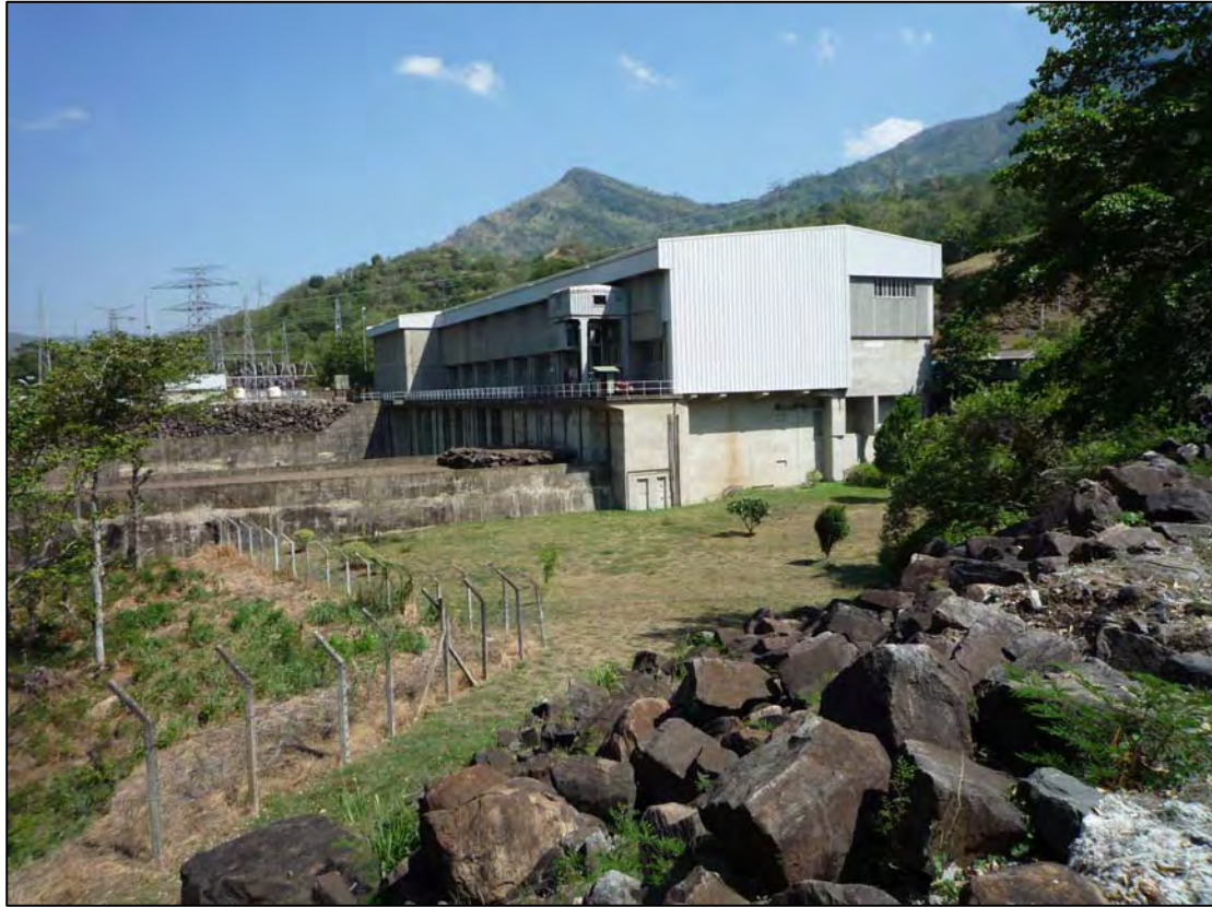
Expansion Area adjacent to Existing Powerhouse
