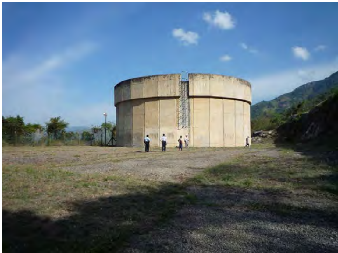
Existing Surge Tank
