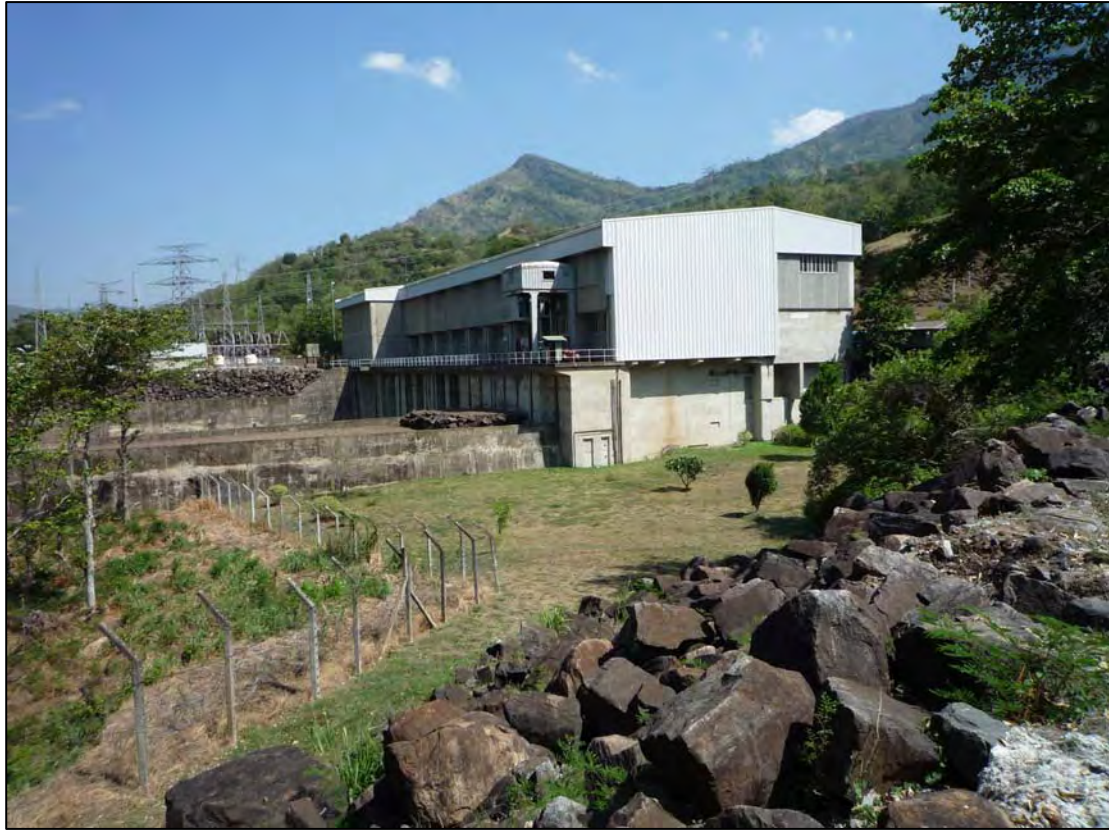
Expansion Area adjacent to Existing Powerhouse
