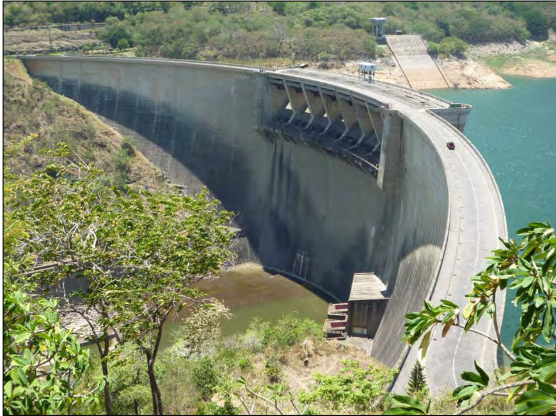
Existing Victoria Dam
