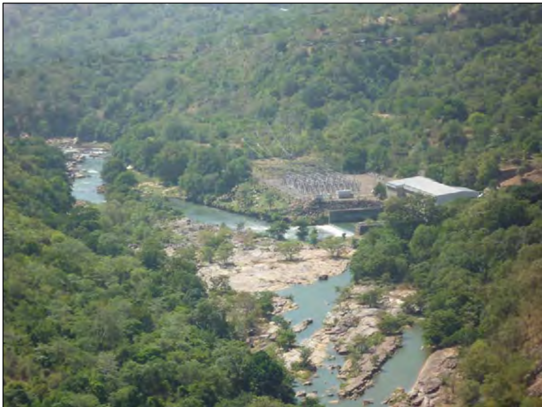
Existing Powerhouse & Switchyard
