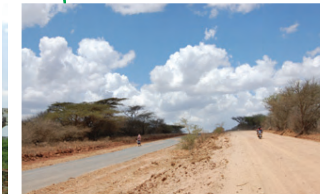
Road Maintenance Site between Nairobi (Kenya) and Arusha (Tanzania)
