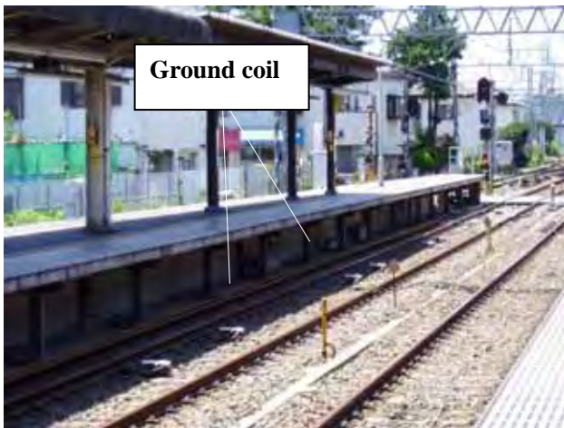
Fig. 5 Ground coils having the speed check function
