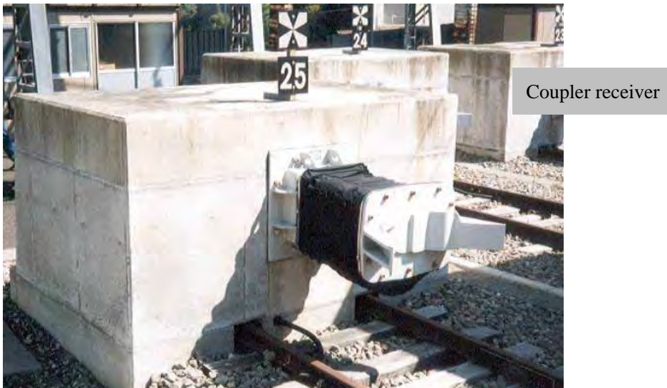
Figure 32.5 Car stop device of hydraulic dumper type
