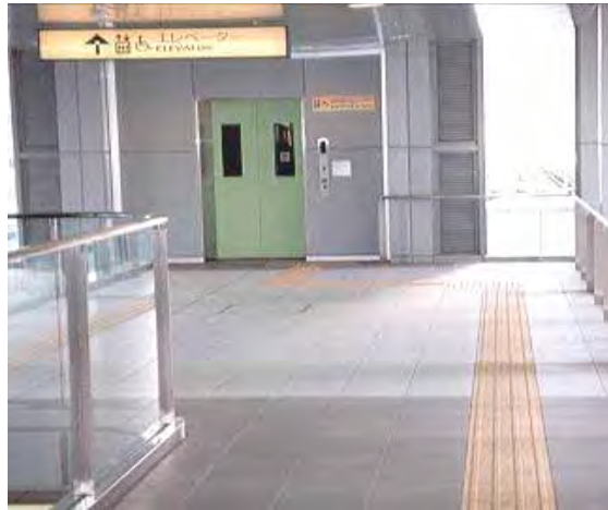
Photograph 1.2. Example of elevator and guidance blocks
