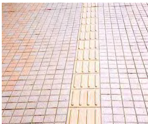
Photograph 1.3. Example of anti slip floor material
