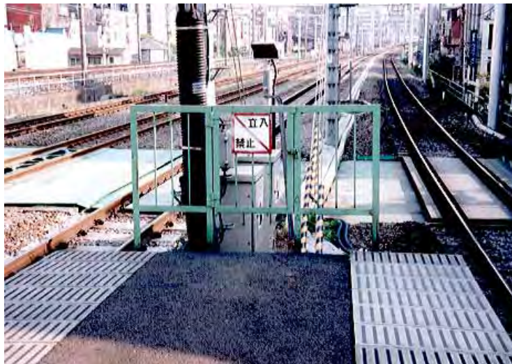
Photograph 38.2 Falling protection fence at the location other than track side
