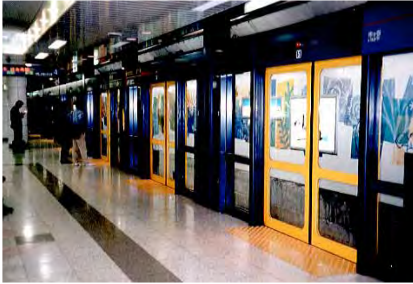
Photograph 38.6 Example of platform doors
