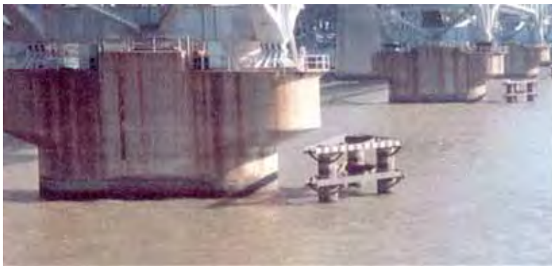
Photograph 31.2 Example of protection work for pier
