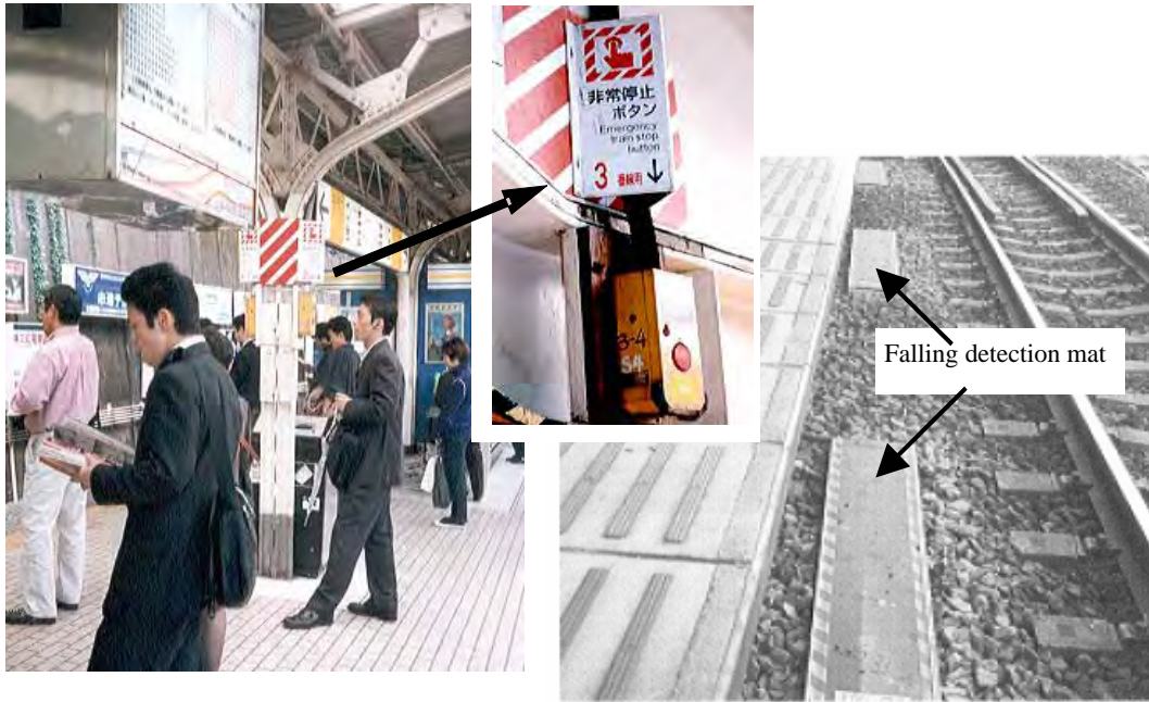
Photograph 38.3 Emergency train stop button
