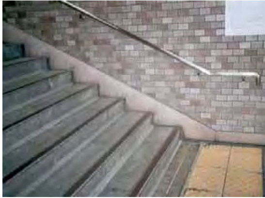
Photograph 1.4. Example of non-slip measure at step edge
