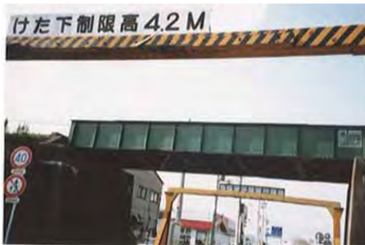
Photograph 31.1 Example of protection work for bridge girder
