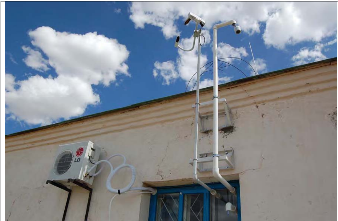
Completion of the Equipment Installation Work at Dalanzadgad Aimag Center 4 September, 2007
