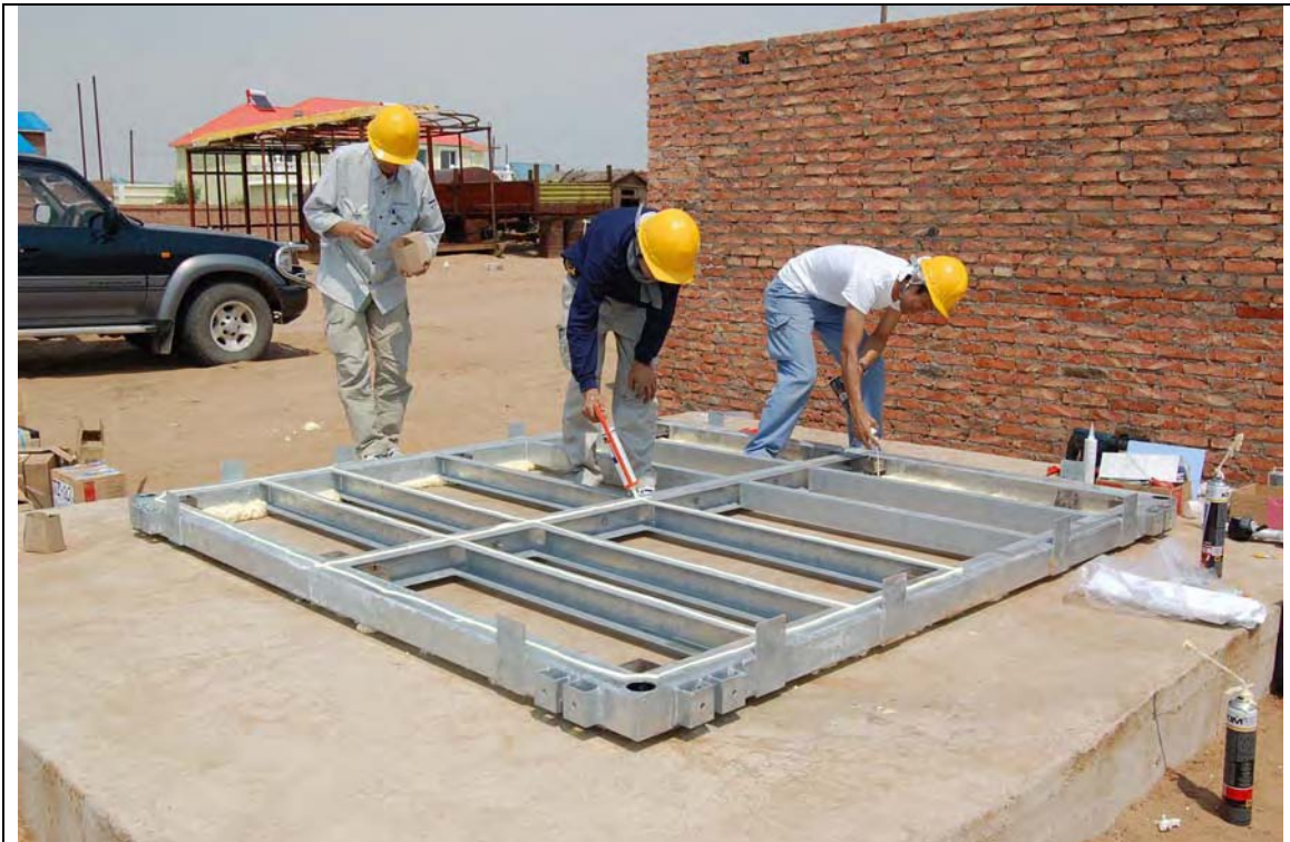
Zamin-ud Meteorological Station (Installation of Container Base) 11 August, 2007
