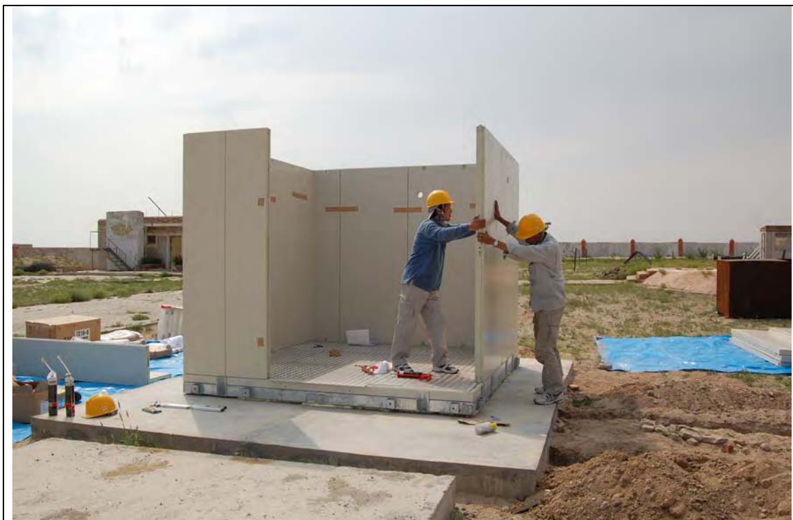
Sain Shand Aimag Center (Assembling Container) 16 August, 2007
