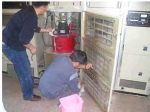
Cleaning of the door of Klystron cabinet
